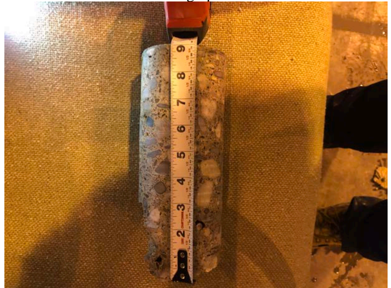
Thickness of cored slab in southern end of building.
