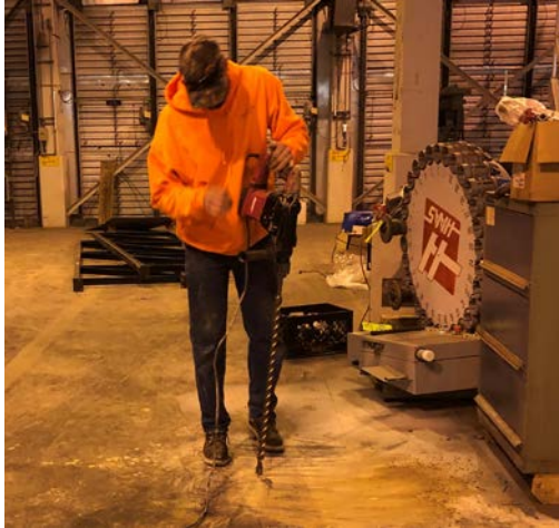
Drilling for monitoring microwell installation.
