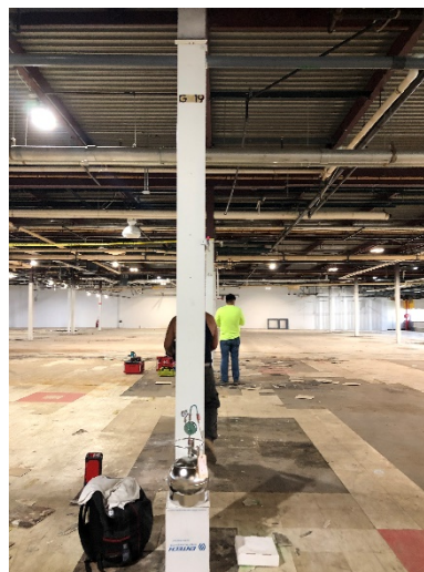
Sample Location IA-8, Column G19 Bldg. 310 (220)
