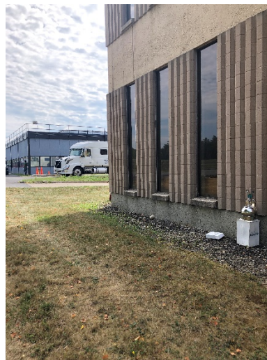
Sample Location AA-1, NE front of Building 320A (210)
