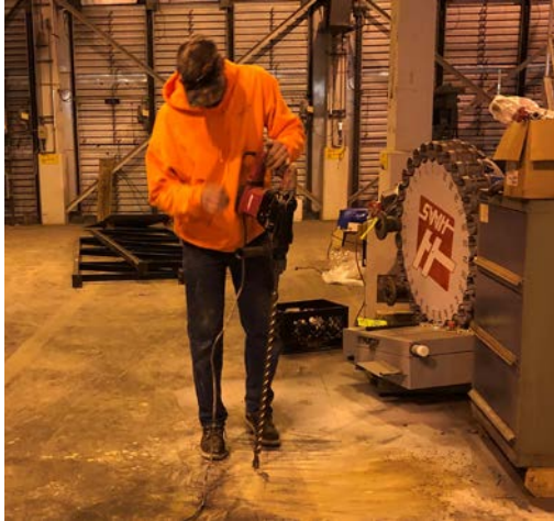
Drilling for monitoring microwell installation.
