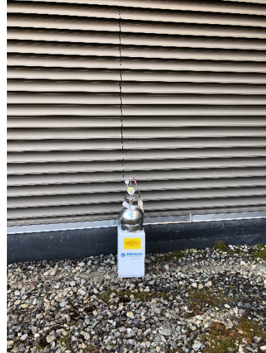
Sample Location AA-01, Rooftop HVAC Unit
