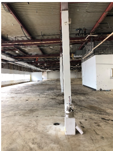
Sample Location IA-6, Column B16 Bldg. 310 (220)
