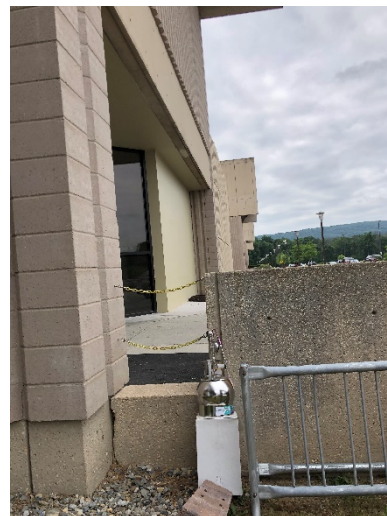
Sample Location AA-1, NW Front of Building
