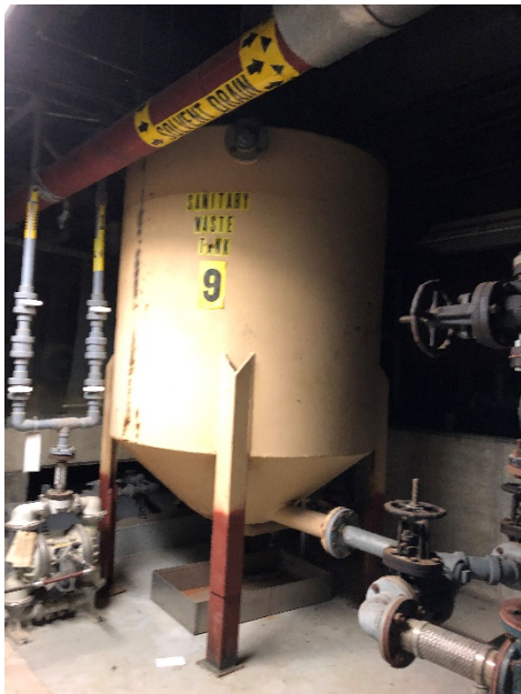
Photo #9: IA-10, Western sub-basement space
