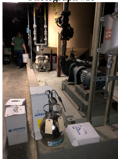
Sample Location IA-10, Western sub-basement space
