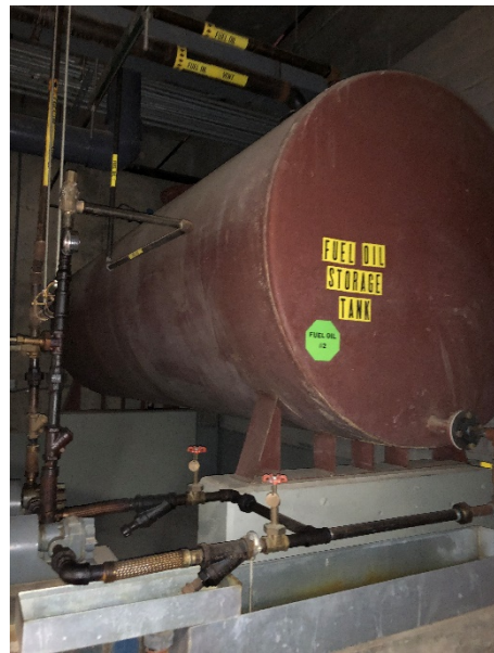
Photo #10: IA-10, Western sub-basement space
