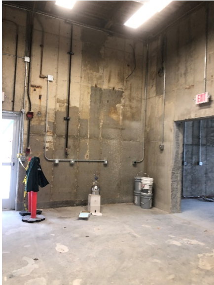
Photograph #5: IA-5 Sampling Location in middle section, kitchen area (Note 4 sealed buckets of paint in the corner of this area).
