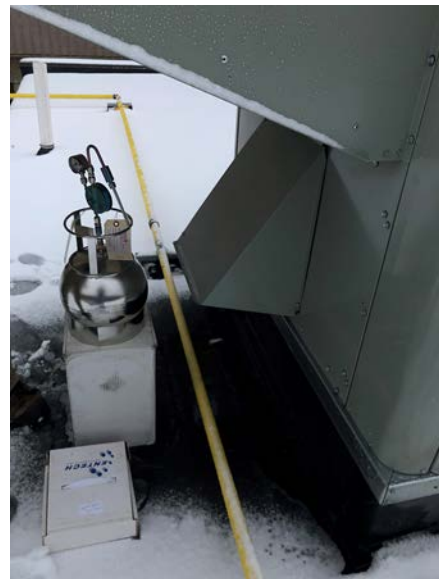
Photograph #8: Ambient Air Sampling Location on roof
