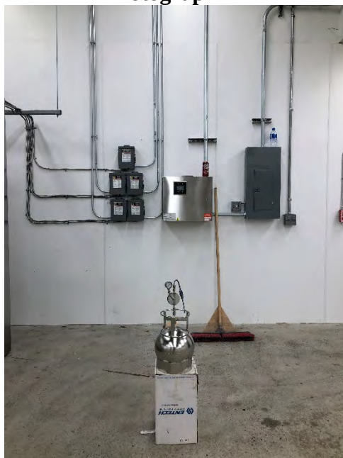
Sample Location SCIA-01, Inside Entrance from Lobby
