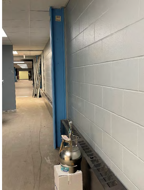
Sample Location IA-02, Hallway
