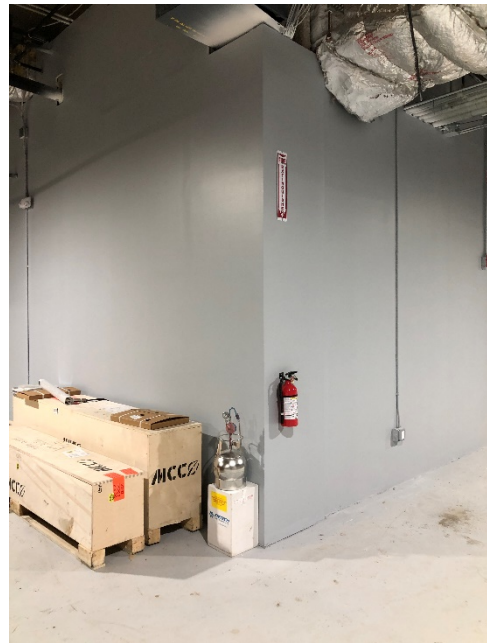
Sample Location MWIA-04, Storage area 1-west
