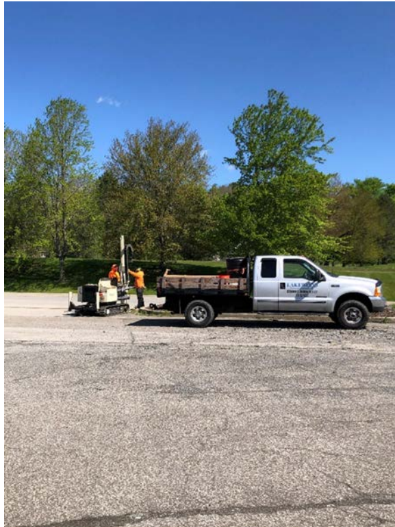
Photograph #2 Lakewood Drilling
