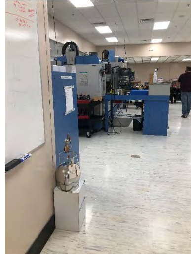
Sample Location IA-3, CNC Machining Center
