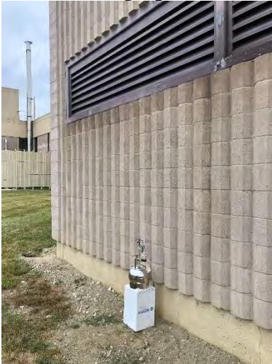
Sample Location AA-1, located Front of Building Under Air Intake for HES
