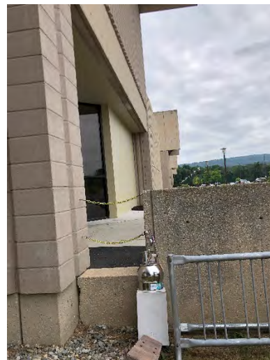
Sample Location AA-1, NW Front of Building
