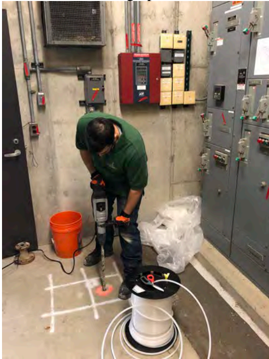
Drilling for monitoring microwell installation in electric room
