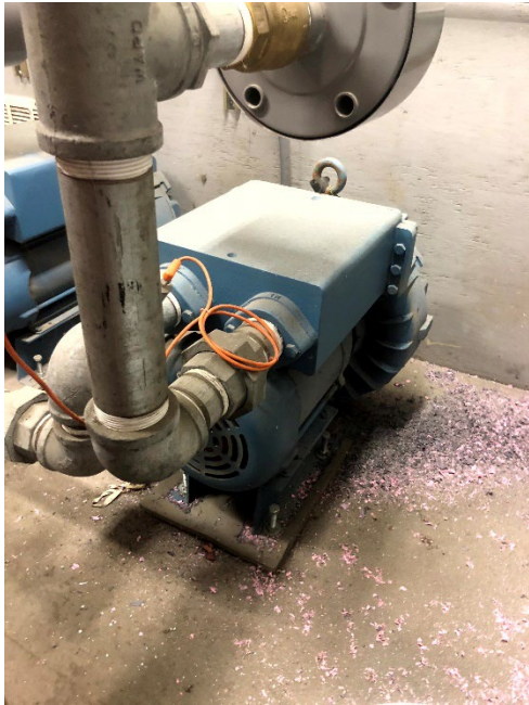
Blower #1 shut off due to banging noise when operating
