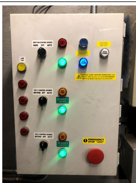
SSDS control box after restart
