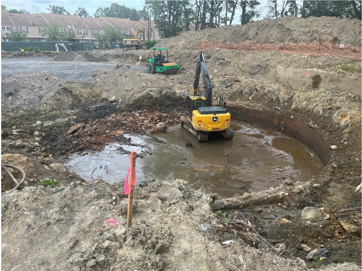
Demolition of the foundation wall.
