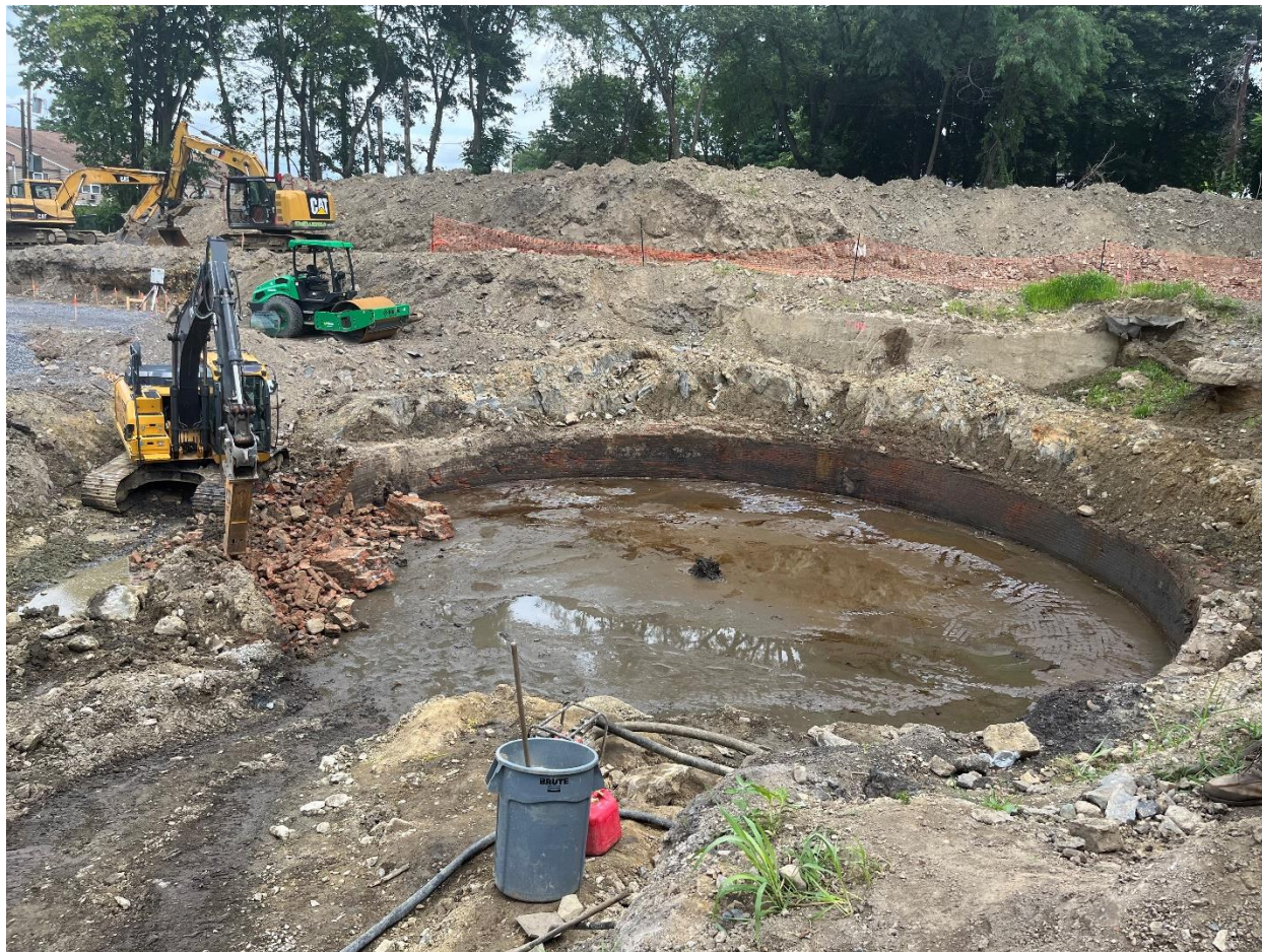
Beginning demolition of the holder's foundation wall.
