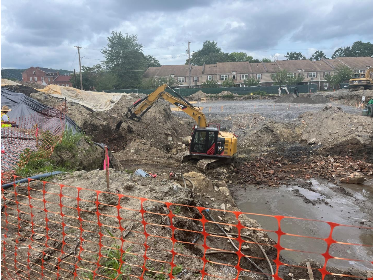
Stockpiling brick from the holder foundation.
