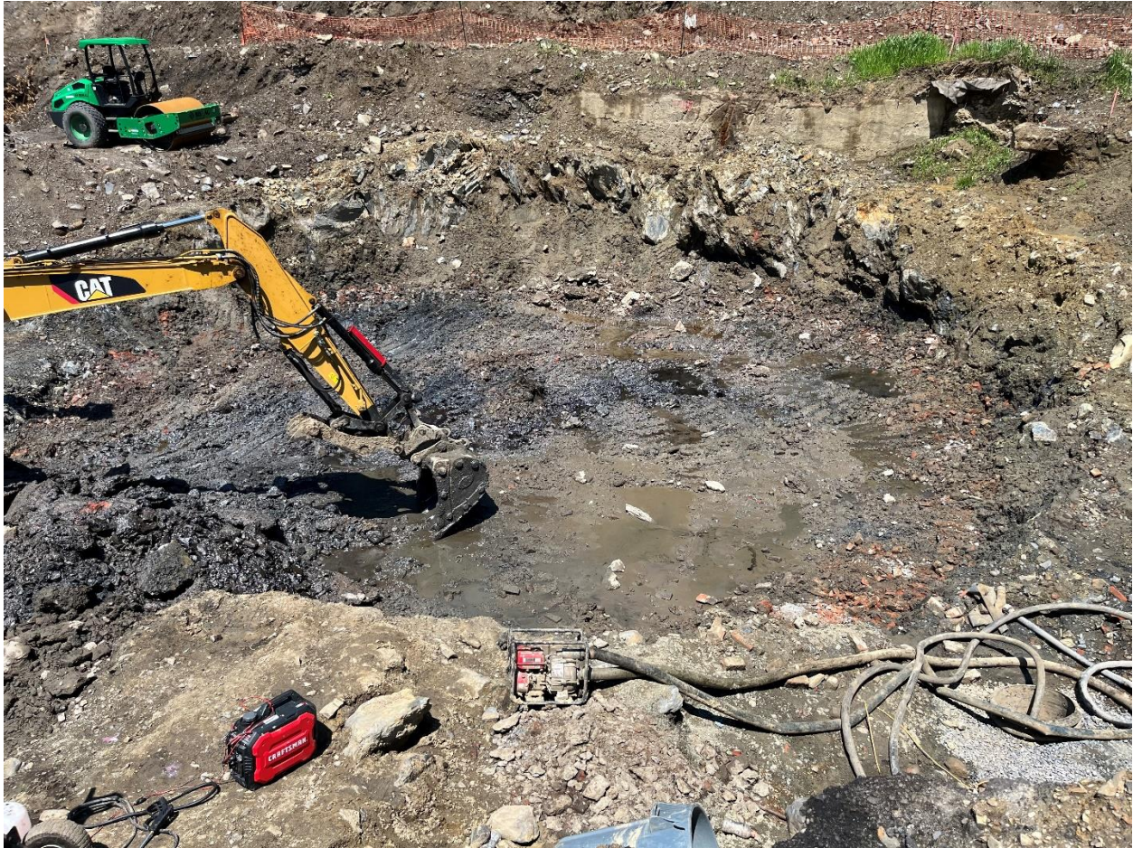
Demolition of the former gas holder floor.
