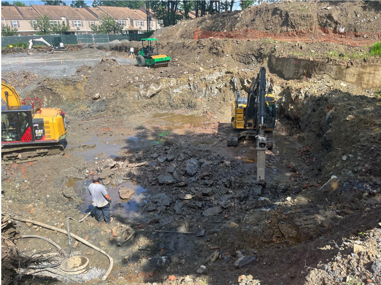
Demolition of the former Gas Holder's floor.
