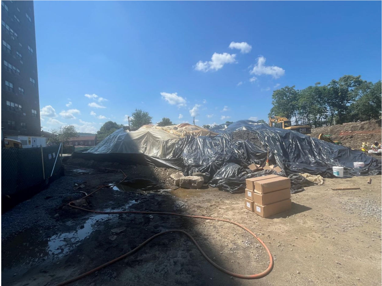
Stockpile covered at the end of the workday.
