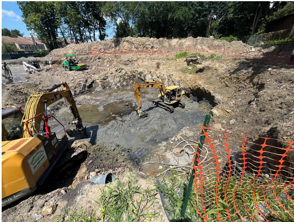
Demolition of the former Gas Holder's floor, facing southeast.
