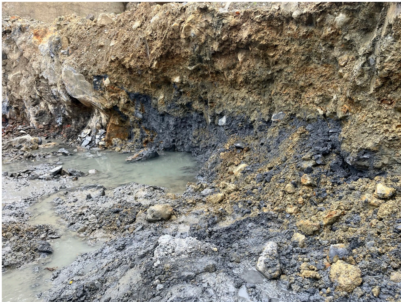
East wall of excavation. One to two foot thick layer of blue stained soil evident just above base of excavation.
