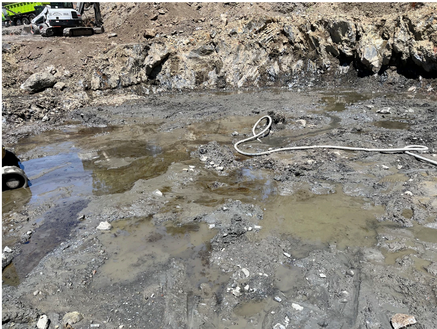
C2G dewatering former holder excavation. Coal Tar blebs and stringers évident in water.
