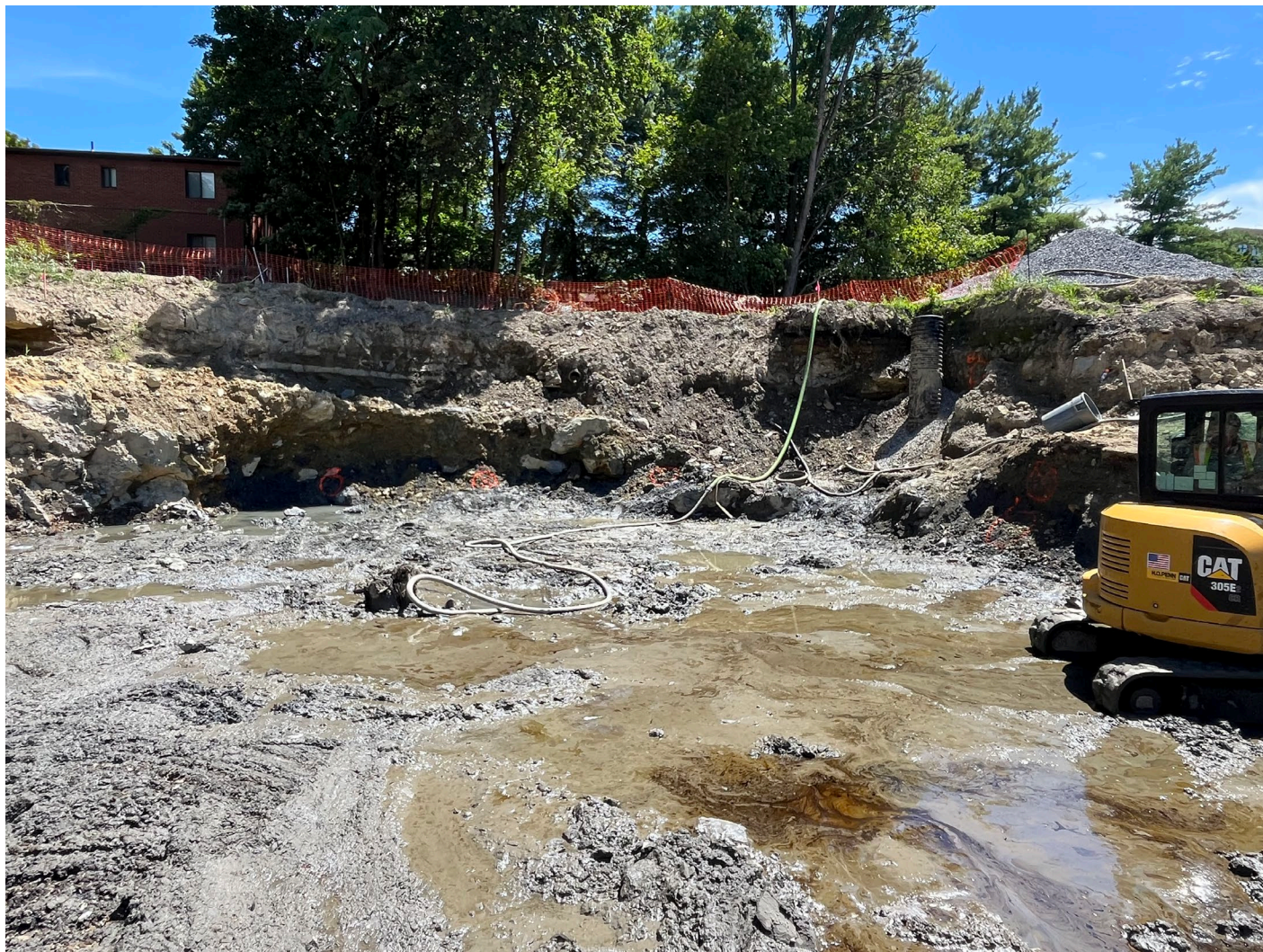
Former holder excavation, coal tar ebullation occuring.
