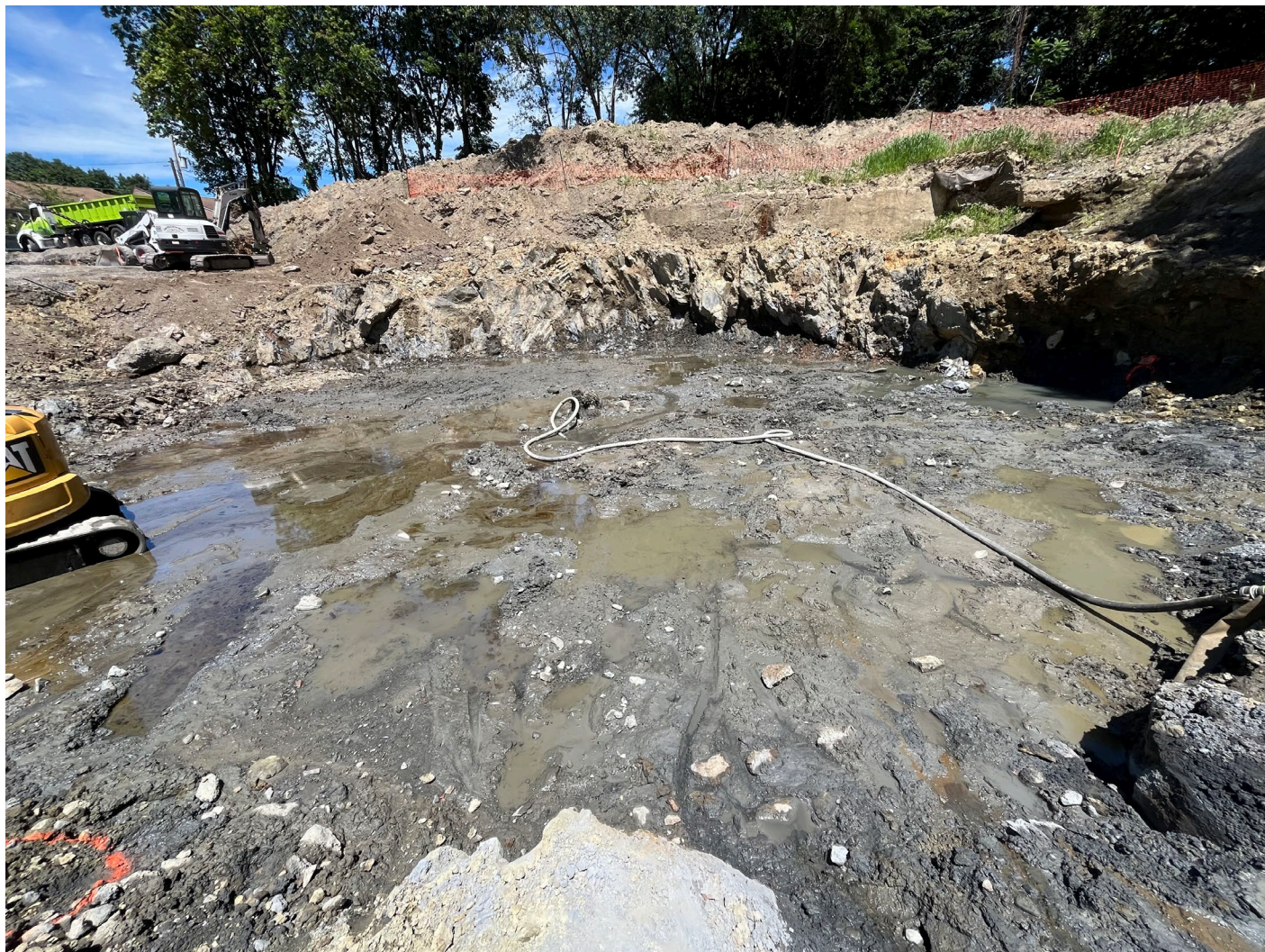
North wall of excavation in background. Second holder foundation on top of bedrock
