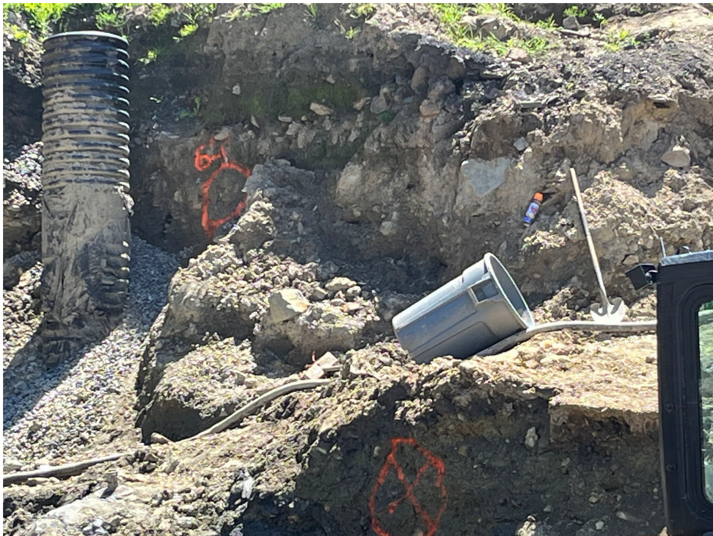
South wall of excavation. Two end point sampling locations marked with orange paint.
