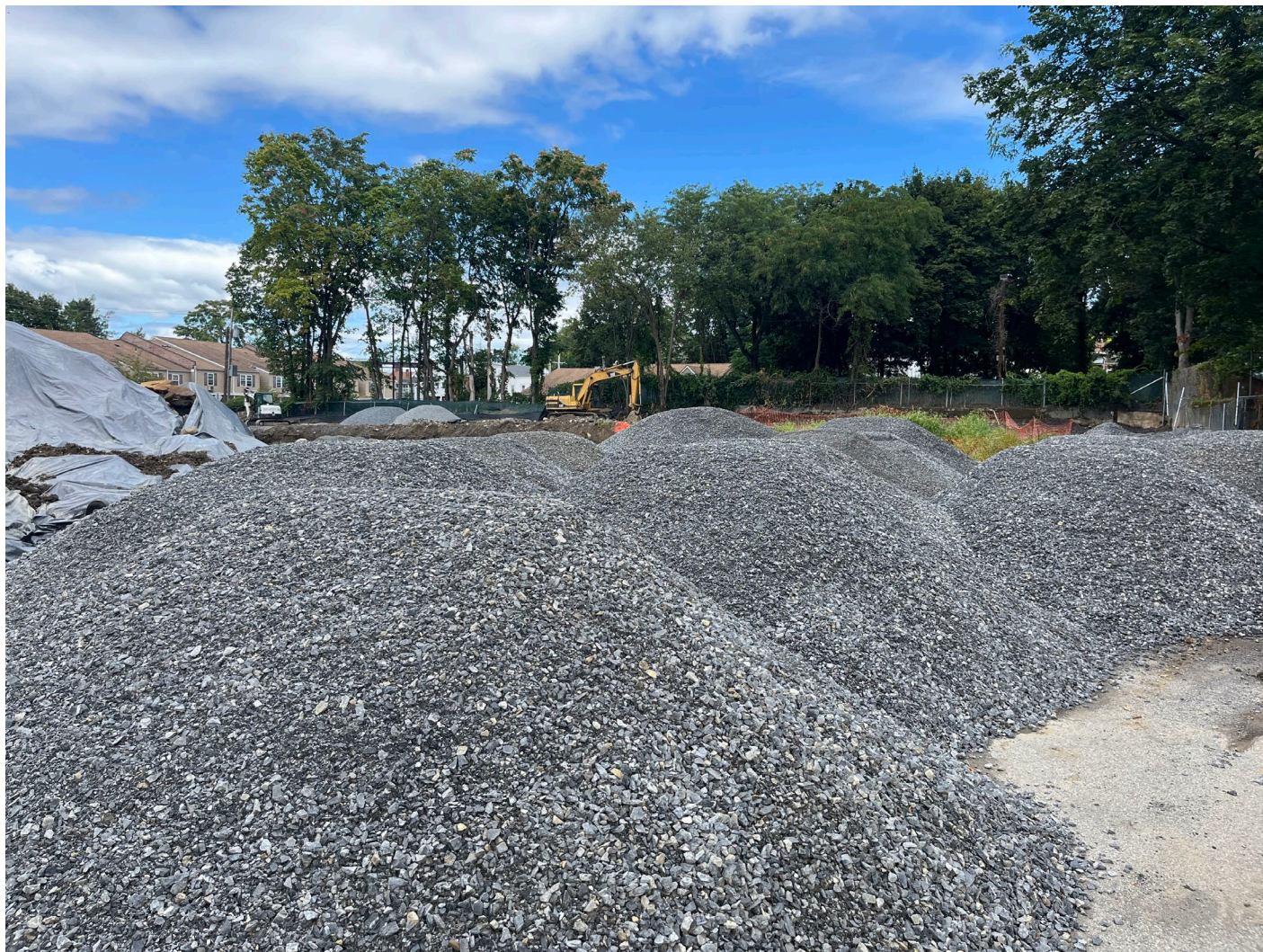
Staged backfill for holder excavation.
