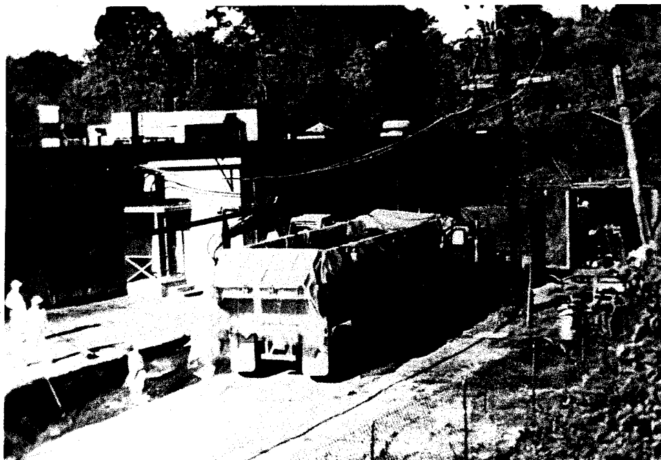
PHOTO 16 HIGH VOLTAGE TRANSFORMERS, POWER LINES AND OVERHEAD UTILITIES IN THE AREA OF EXCAVATION. THESE UTILITIES WERE ALSO VERY LOW.
