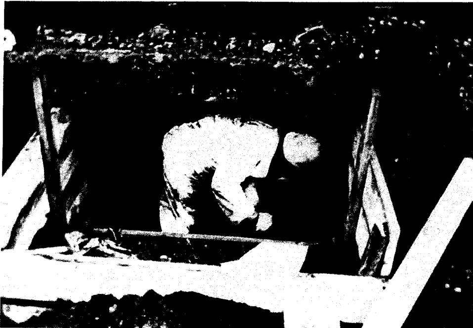
PHOTO 30 FOOTING SUPPORT CONSTRUCTION UTILIZING HAND DUG WOOD FRAME SLIP FORMS
