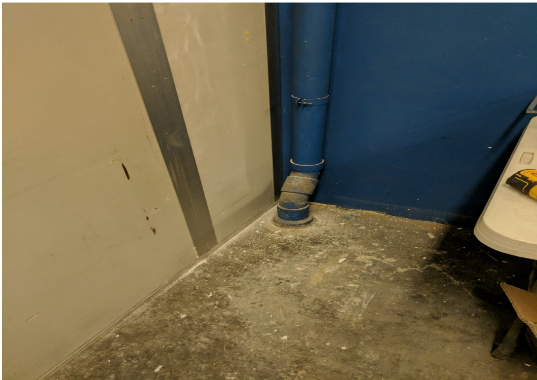
Photo 6: Interior riser joint at concrete floor 2/1/19
