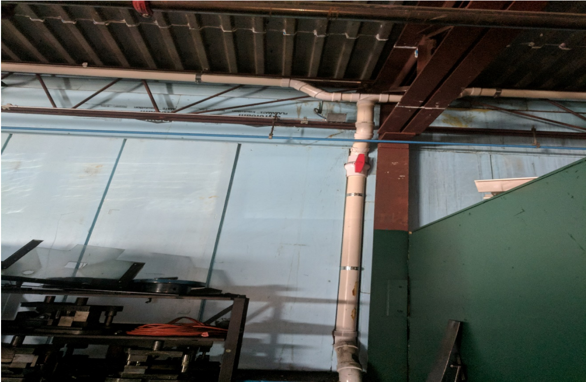
Photo 7: Interior riser and junction at pipe typical 2/1/19
