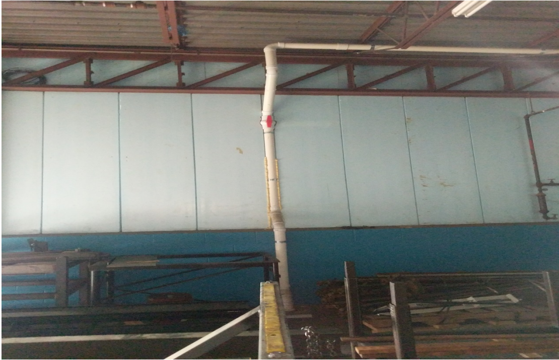
Photo 1: Interior PVC riser showing typical open valve 2/1/19
