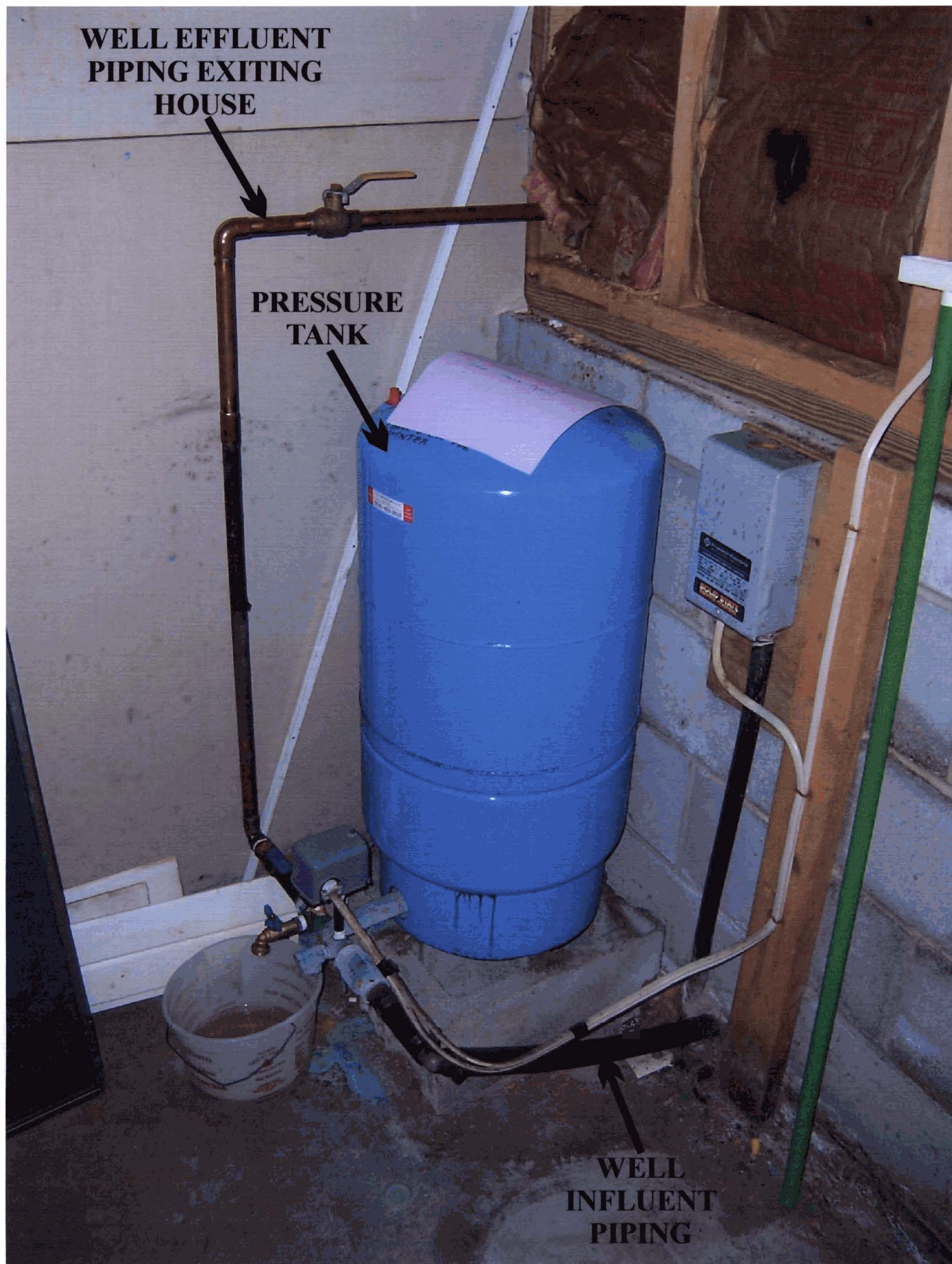
View of supply well influent piping, pressure tank, and well effluent piping. 9-7-07.
