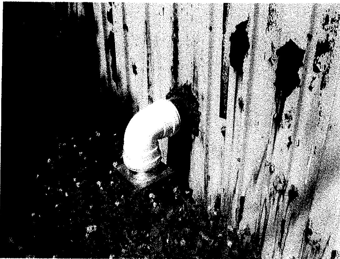
External portion of blower air influent pipe. 5/21/07.
