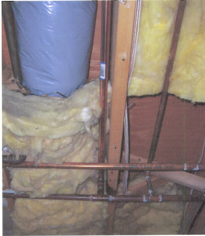
Connection of new municipal piping into existing indoor piping in basement of Lot 9. 10-3-08.
