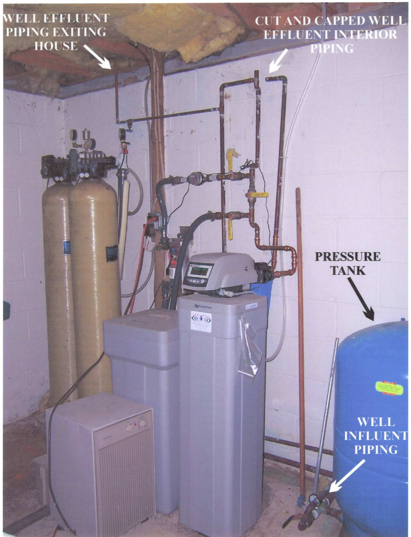
View of supply well influent piping, pressure tank, and well effluent piping in basement of Lot 9. 10-3-08.
