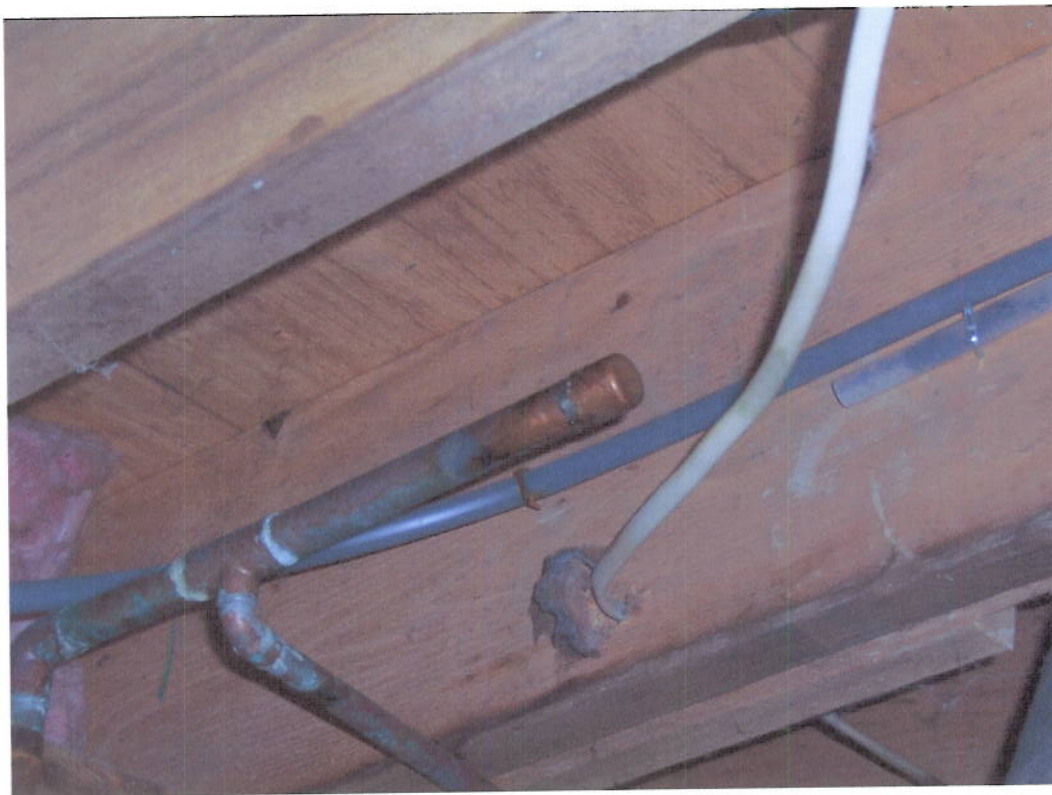
Cut and capped interior well line piping in basement of Lot 10. 9-30-08.
