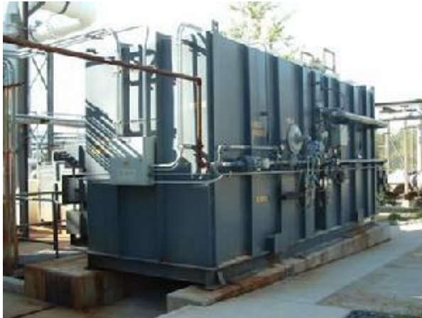
AL6XN 8,000 SCFM RETOX RTO-REACTOR VENTS
