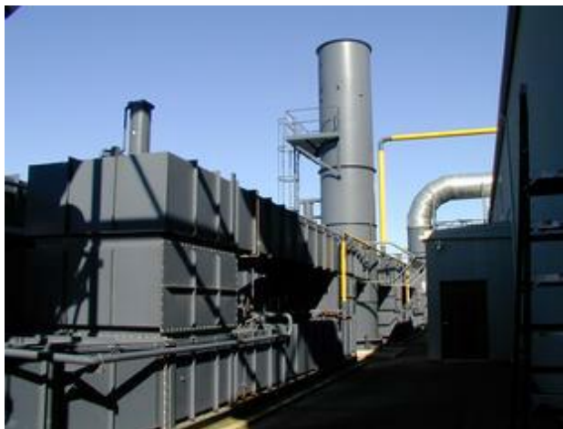
2 Module RETOX LFC RTO System-120,000 SCFM Total for Paint Finishing Spray Booths
