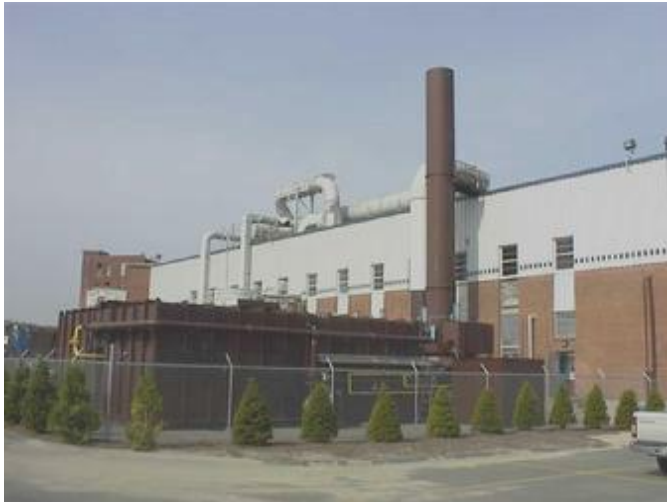
RETOX 62,000 SCFM LFC RTO-WEB CONVERTING & PRINTING-REPLACED CARBON SOLVENT RECOVERY UNIT
