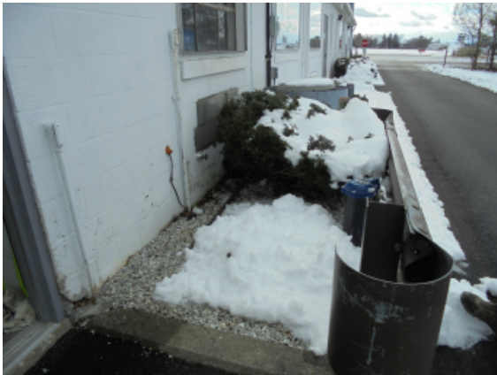
Entrance to boiler room at former IBM hangar
