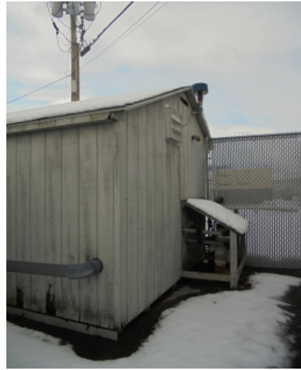
Former treatment system building at flagship hangar
