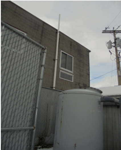
Former treatment system at Flagship hangar
