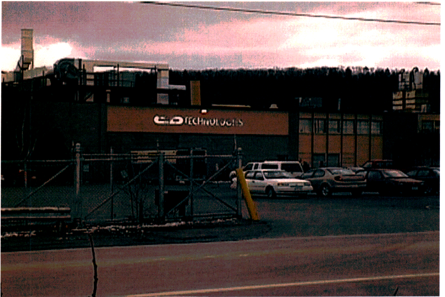
C&D Facility from Route 209 Entrance
