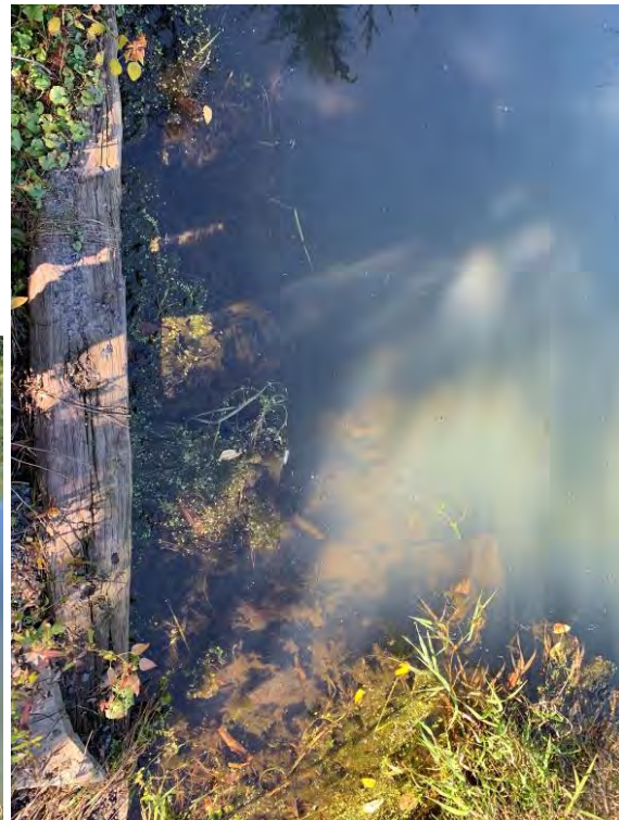
Upstream mouth of Swartwout Road culvert. Dense woody debris and mud covered the culvert opening. Culvert showed no evidence of recent disturbance – fill over culvert was not appreciably different from adjacent roadway.
