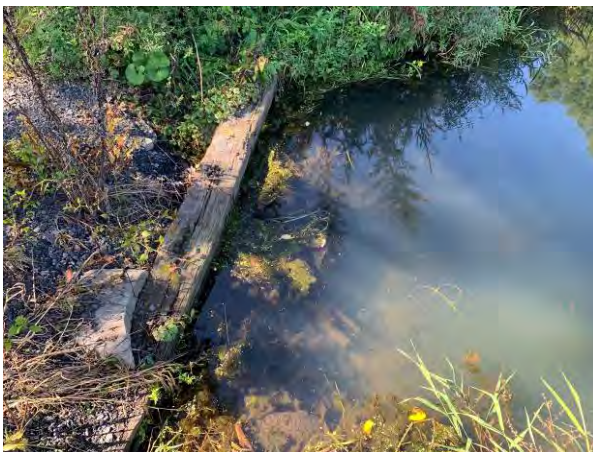
Upstream mouth of Swartwout Road culvert. Dense woody debris and mud covered the culvert opening. Culvert showed no evidence of recent disturbance – fill over culvert was not appreciably different from adjacent roadway.
