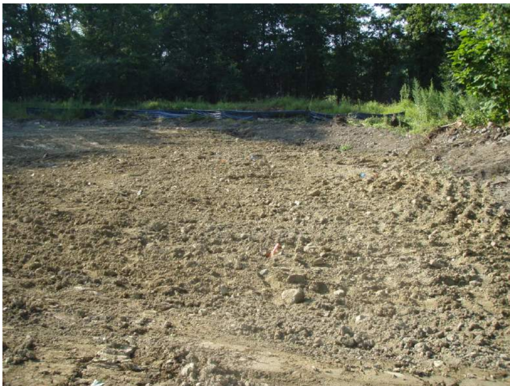
Silt fence on the southwestern side of the Land Spreading Area excavation.
