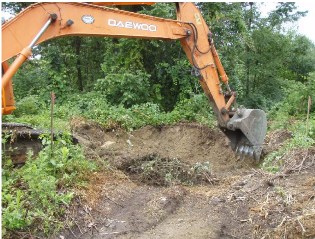
Excavation of soil with a concentration > 1,000 ppm chromium from the Soil Consolidation Area. Extent of the area to be excavated was marked by upright wooden stakes.
