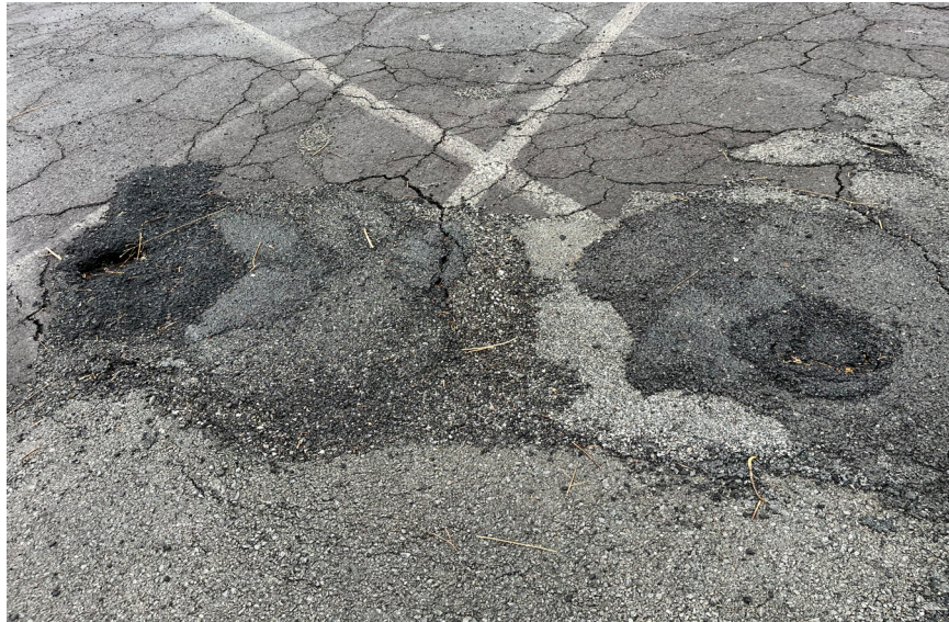
Photograph 5 Representative Parking Lot Photograph Showing Areas of Repair
