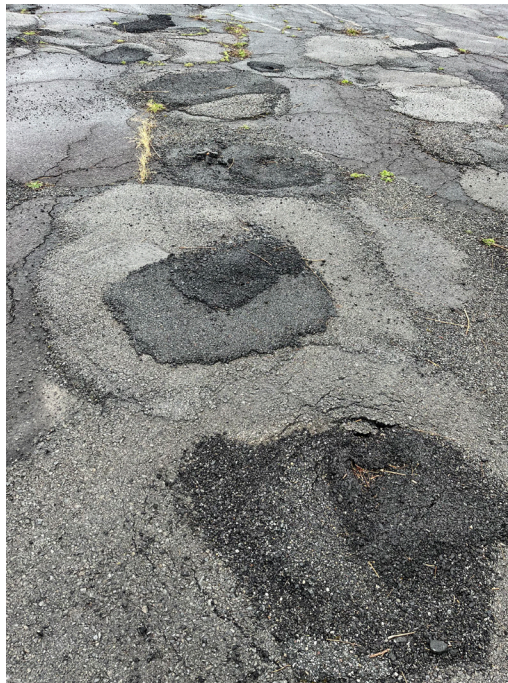
Photograph 6 Representative Parking Lot Photograph Showing Areas of Repair
