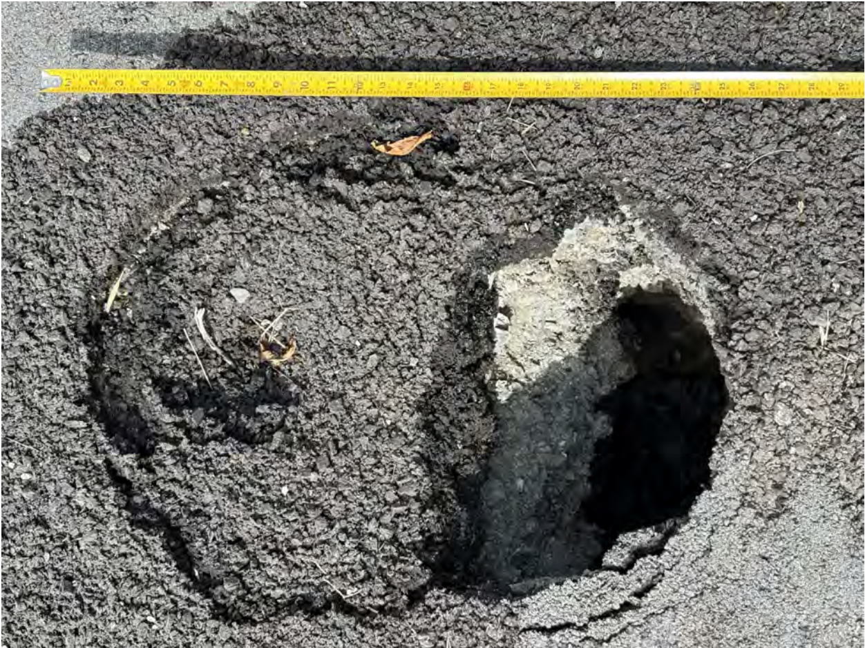
Photograph 5 Representative Parking Lot Photograph Showing Areas of Repair
