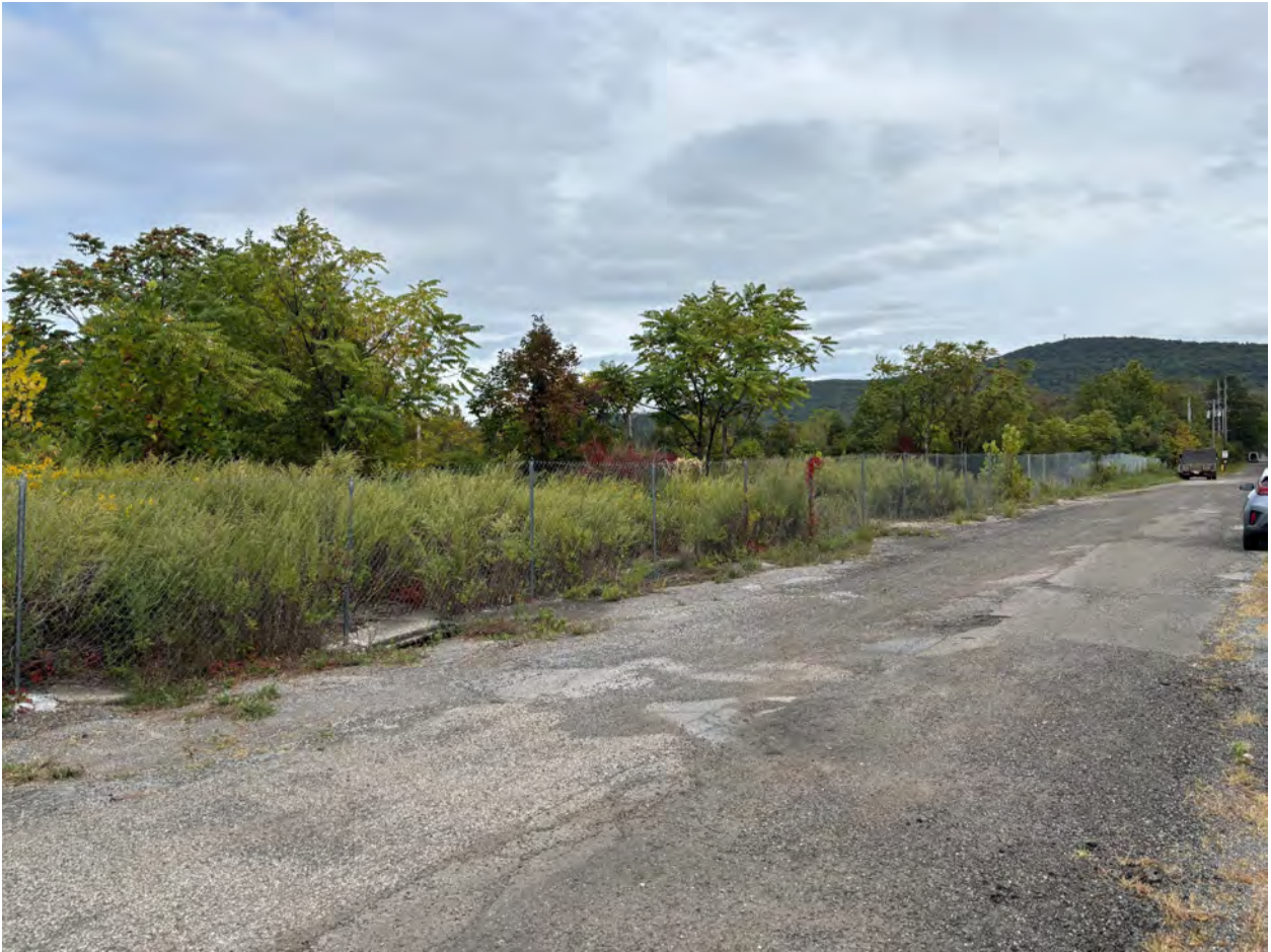
Photograph 1 Parking Lot Fence Facing Southwest
