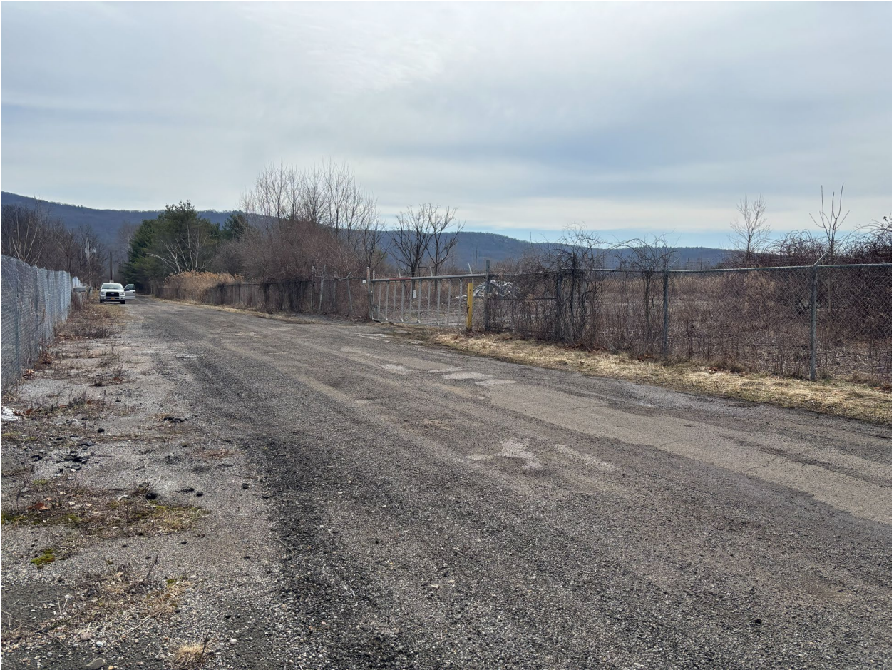
Photograph 2 Lot Fence facing Southeast
