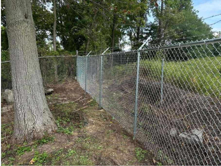
Photo 23: Northwestern corner of site following fence replacement
