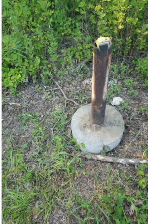
Photo 5: Monitoring Well LF-16S prior to repairs
