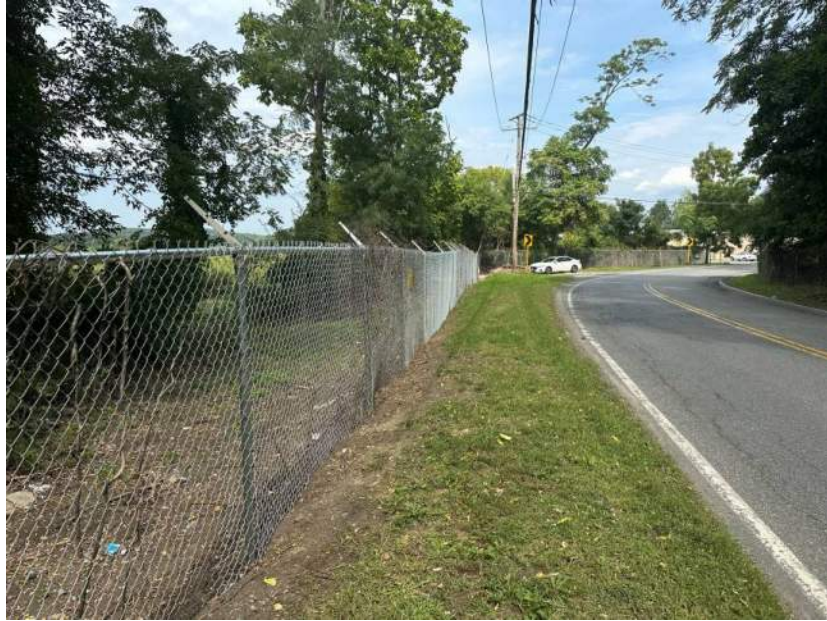
Photo 13: Fence along Pierces Road showing completed repairs
