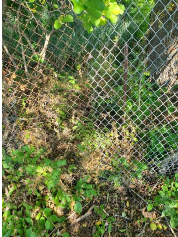
Photo 15: Fence along northern site border after repairs were completed
