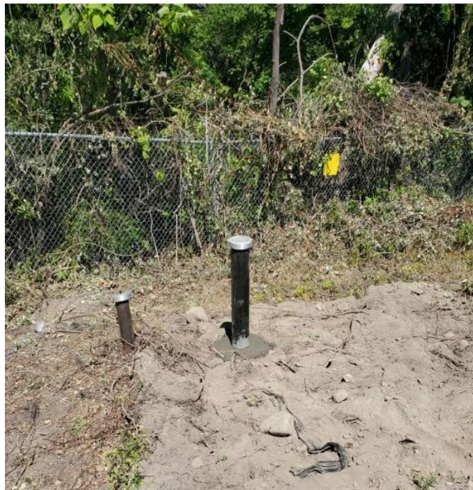
Photo 4: Monitoring Well LF-15S after stickup and pad replacement
