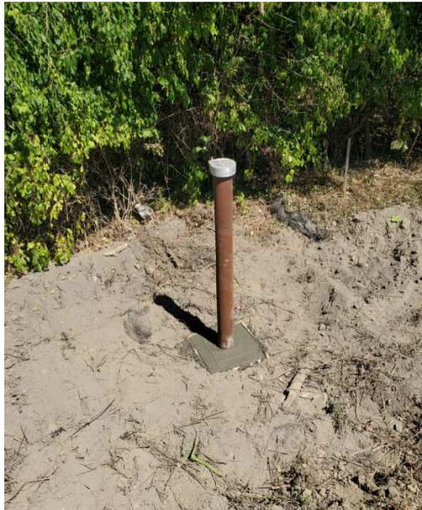
Photo 2: Monitoring Well LF-17D after stickup and pad replacement. Mulching and reseedling of disturbed areas will occur in October
