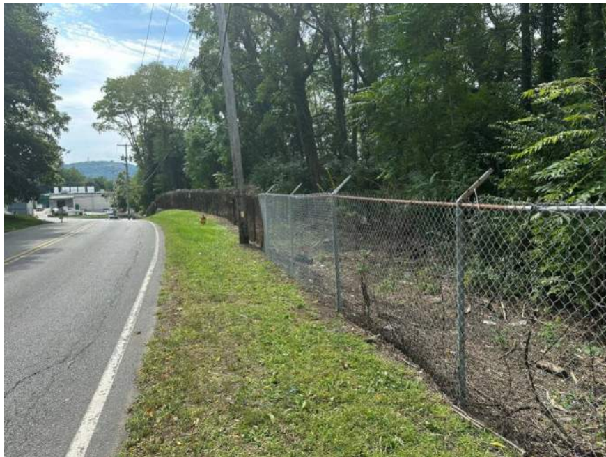
Photo 12: Fence along Pierces Road showing completed repairs
