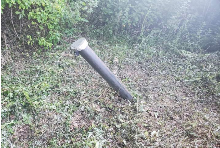
Photo 1: Monitoring Well LF-17D prior to repairs
