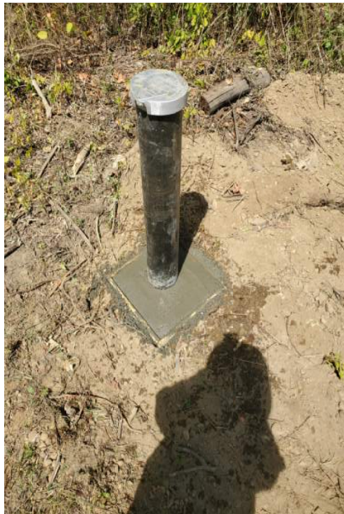
Photo 6: Monitoring Well LF-16S after stickup and pad replacement
