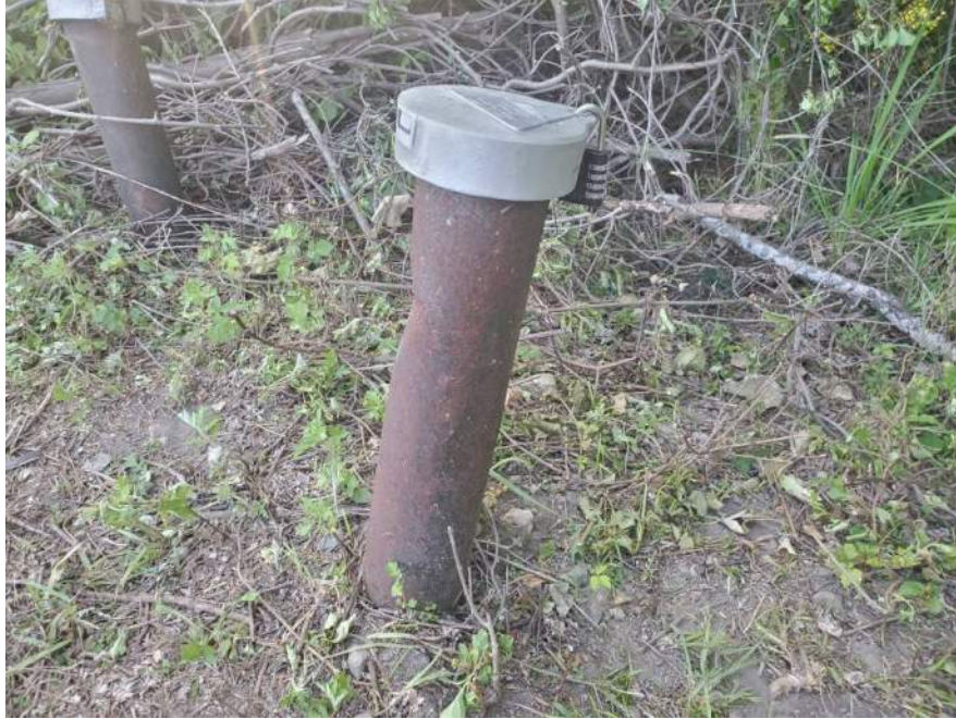
Photo 3: Monitoring Well LF-15S prior to repairs
