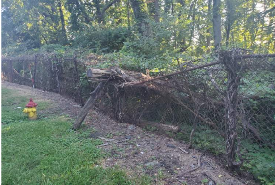
Photo 9: Fence along Pierces Road prior to repairs
