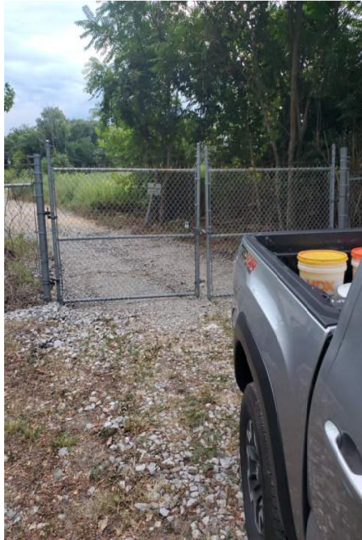
Photo 11: Gate along Pierces Road after repairs
