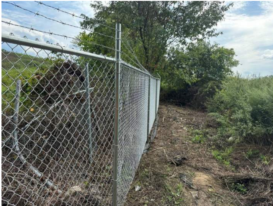
Photo 24: Northwestern corner of site following fence replacement
