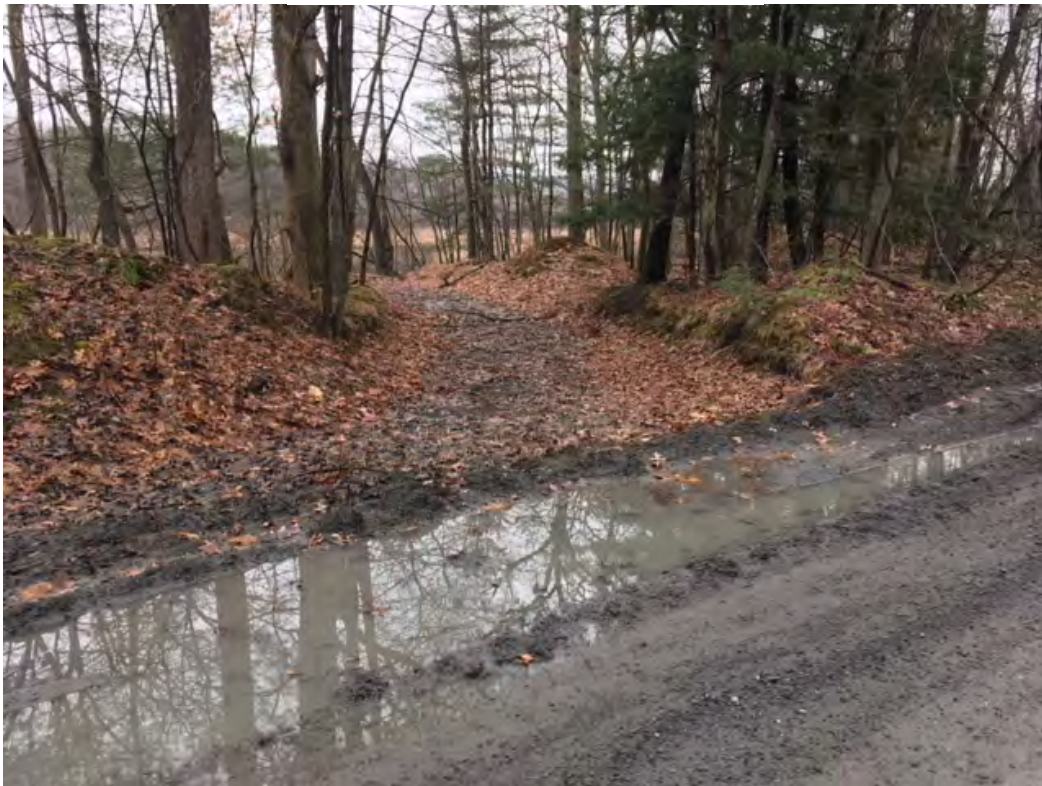
Drainage from quarry road to Gold Creek
