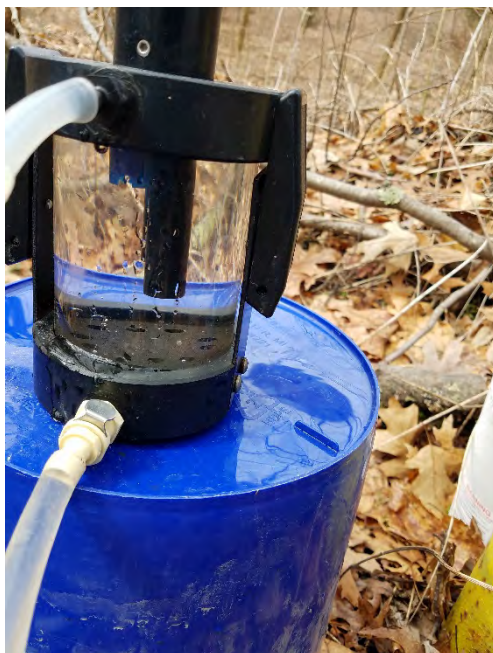
Clear water during purging of monitoring well
