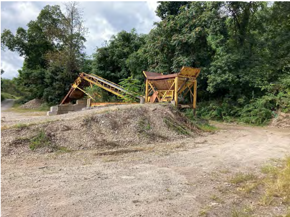
Screening plant for City of Port Jervis sand and gravel operation
