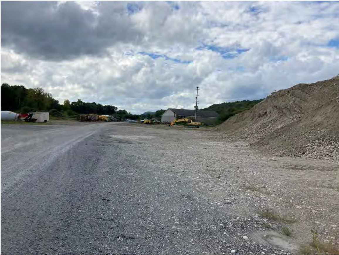
A truck yard, garage, and gravel storage areas for Dick's concrete are located southwest of the C&D site
