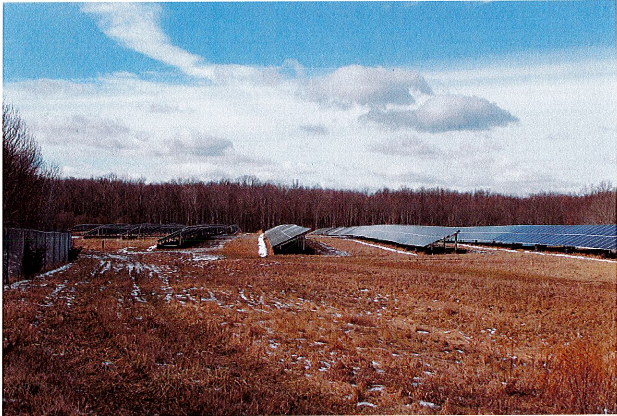
#3 View South of South Cell
