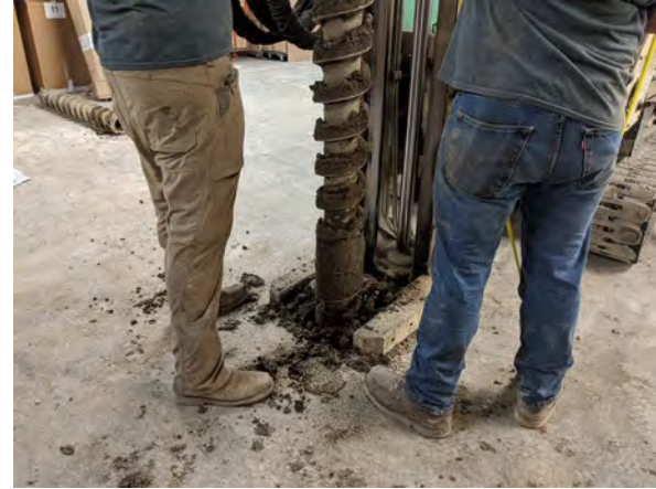
6. Over drilling boreholes with auger
