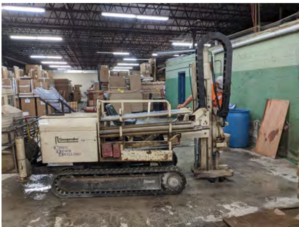
3. Advancing soil borings
