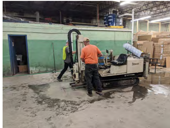
2. Preparing to breaking concrete with rotary hammer
