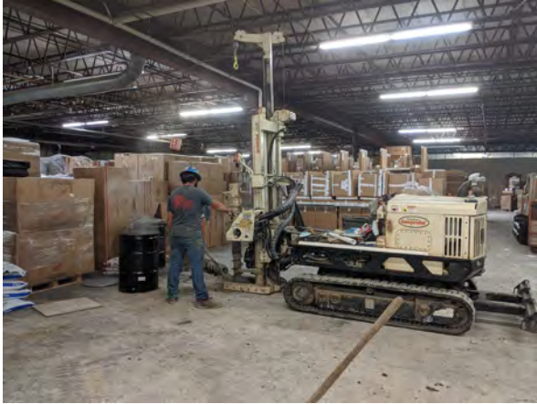
5. Over drilling boreholes with auger
