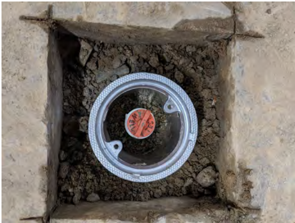
7. Newly installed well
