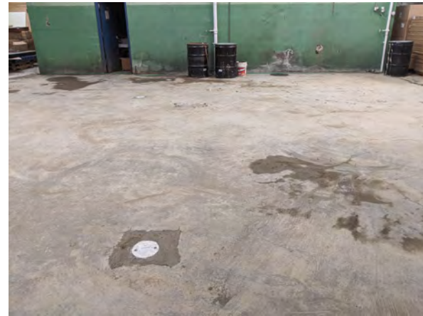
8. Well finished flush with concrete slab
