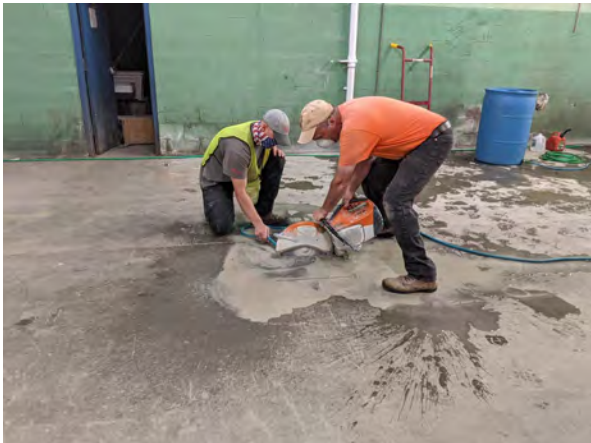
1. Cutting floor slab
