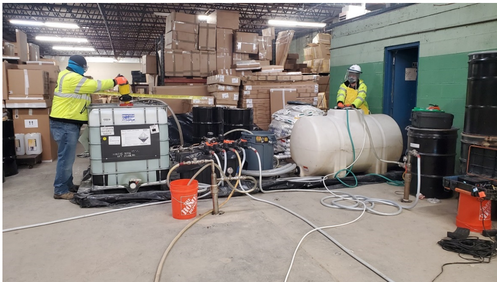
Photograph 10. MECx transferring NaOH solution to mix tank for injections.
