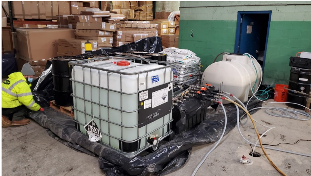
Photograph 4. NaOH staged within containment.
