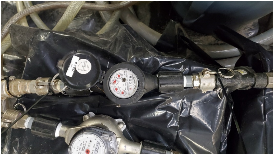
Photograph 11. MECx changed out totalizer flowmeter because original unit stopped working.
