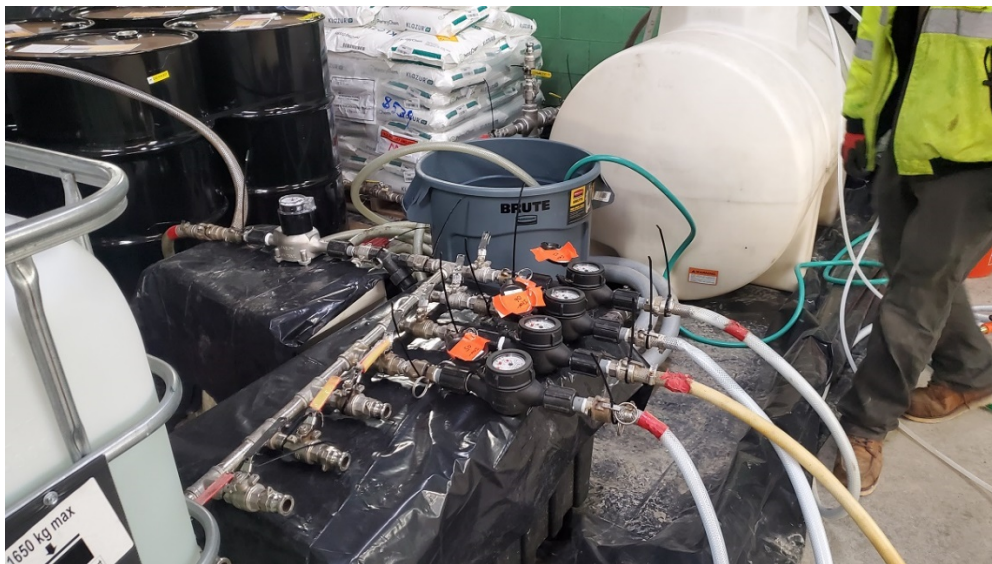
Photograph 6. Flow meters set up at manifold to monitor flow rates and totals of injections during ISCO injections.
