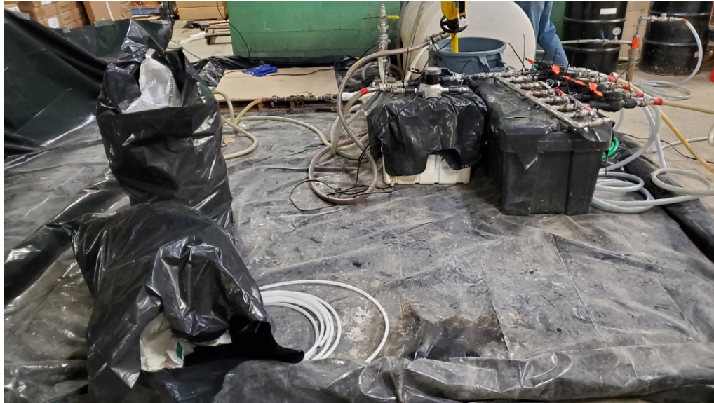
Photograph 15. Containment area cleared of empty containers and equipment during the injection of the last batch of PeroxyChem Klozur® SP.
