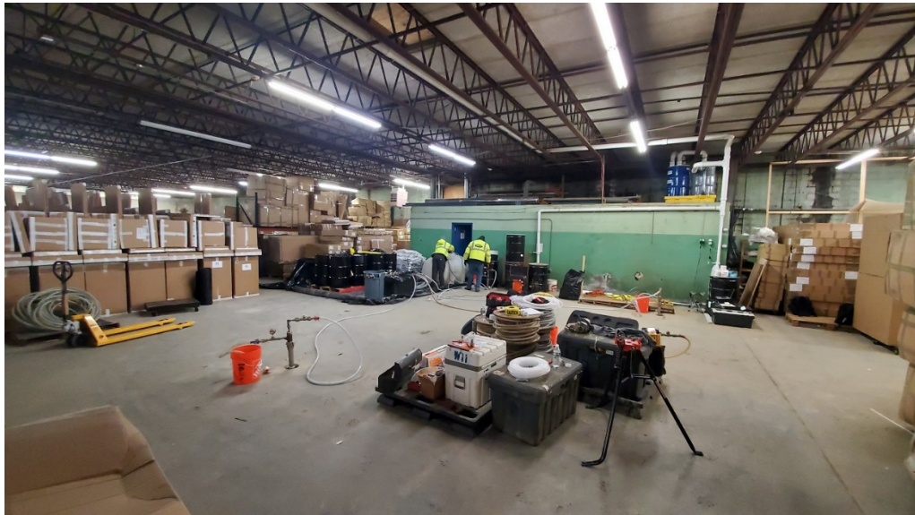
Photograph 1. Remedial action area during setup of ISCO injection equipment, view toward the southwest.
