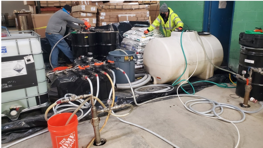
Photograph 9. MECx transferring d-limonene to mix tank with drum pump.
