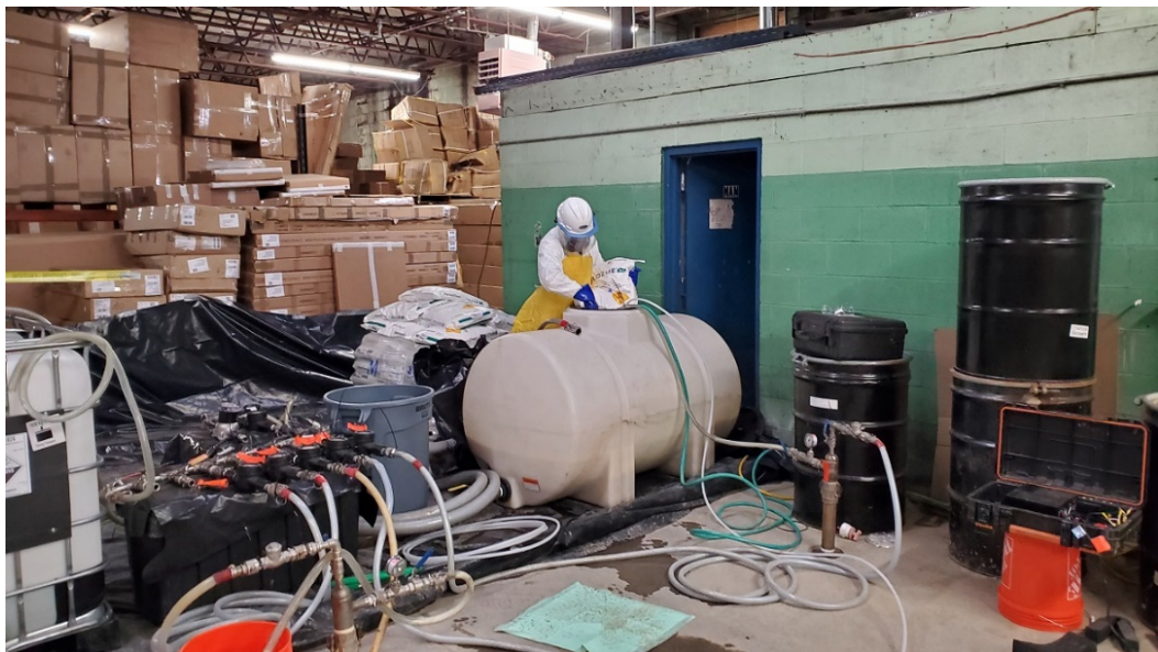
Photograph 12. MECx begins to mix PeroxyChem Klozur® SP in mix tank for injections.
