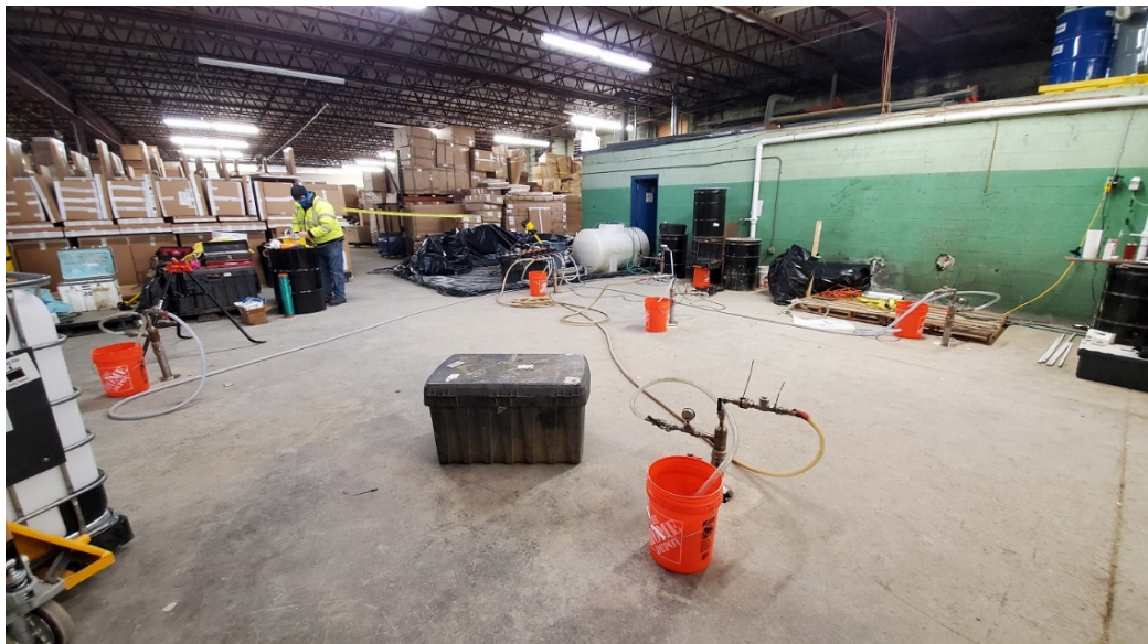
Photograph 14. Overview of RA area with ISCO injections running at all 6 wellheads.
