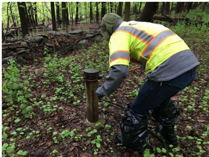
Photo 5: Looking east at well BR-3. Locks on all wells were rusted closed and needed to be cut and replaced. New locks are Master Lock® with key code 2537.
