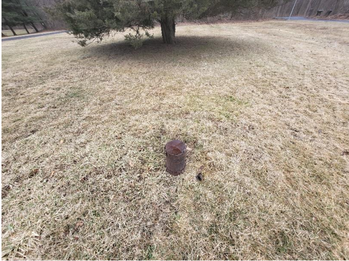
Photo 1: Photograph of an old/not in use well located in the front yard of 94 Peddler Hill Road, casing was rusted and well was in poor condition. Facing southeast.
