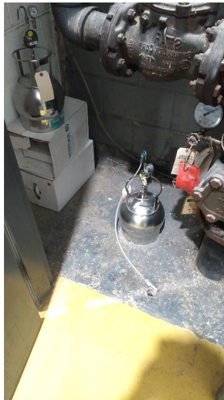
Photograph 4: SS-SV-06 not connected to subslab at test completion.
