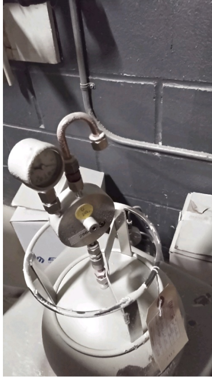
Photograph 5: SS-IA-04 dusted when test completed (Garbage Room).
