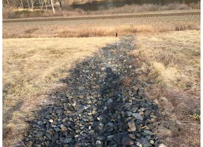
**Photo 6:** Looking east. View of drainage swale on eastern slope of landfill.
