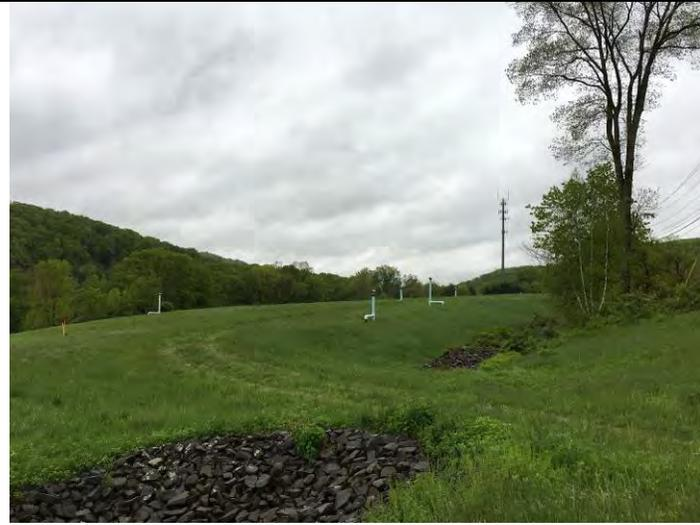
**Photo 3:** Looking south. View of the landfill cap and gas monitoring vents.
