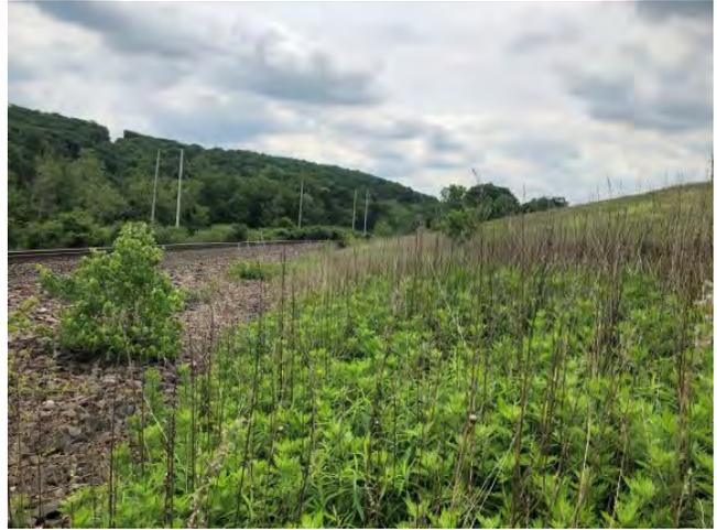
**Photo 2:** Looking south. View of the high vegetation (both alive and dead) located in all of the drainage swales.
