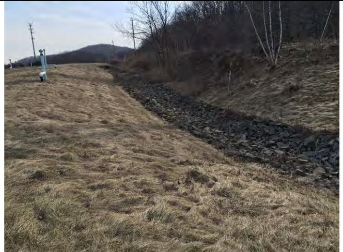
**Photo 4:** Looking south. View of drainage swale on the western side of the site.
