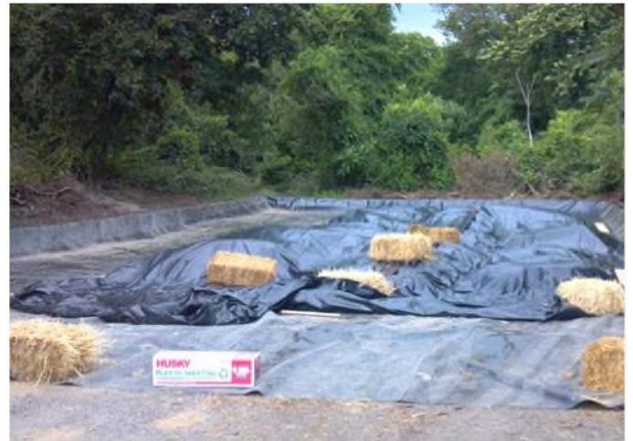
Photo 3 – Stockpiled soil covered to protect from rain
