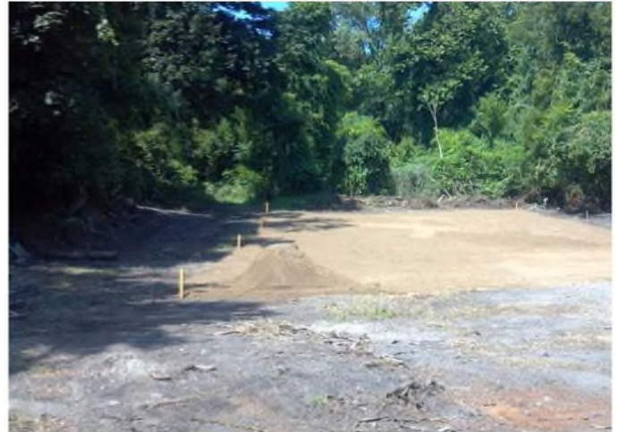
Photo 1 – Preparing lined staging area
