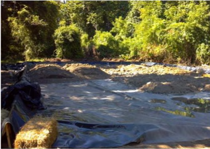
Photo 4 – Soil in windrows for exposure to air
