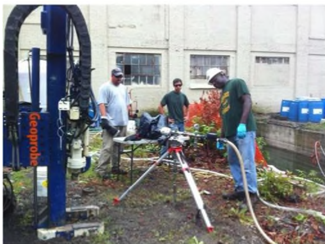
Photo 6 – Injecting persulfate
