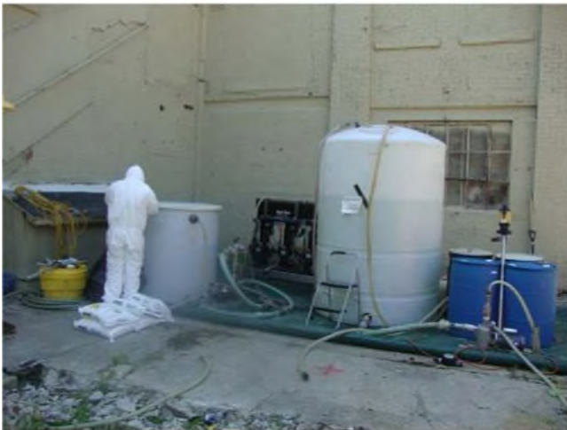
Photo 2 – Mixing sodium persulfate for injections
