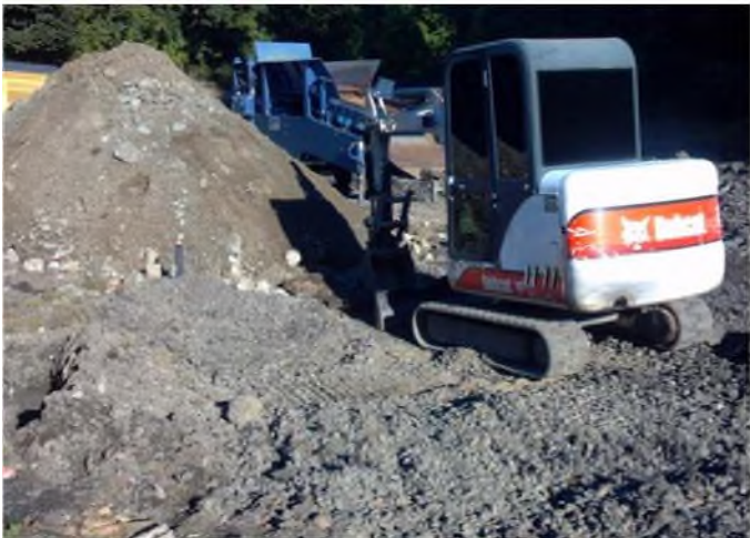
Photo 10 – Loading soil into screener
