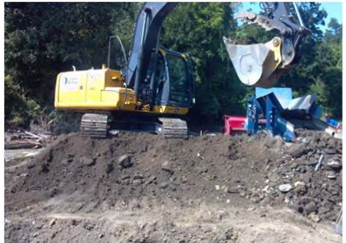
Photo 11 - Loading soil into screener
