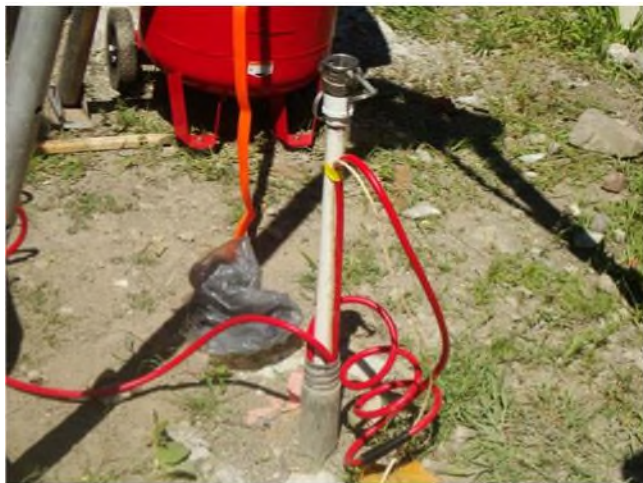
Photo 4 – Inserting injection tool into well
