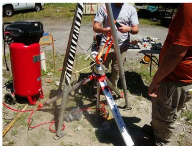
Photo 7 – Injecting persulfate
