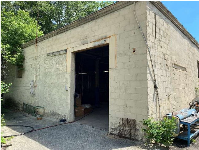
Photo 7. Piano Felt Bldg. entrance.
