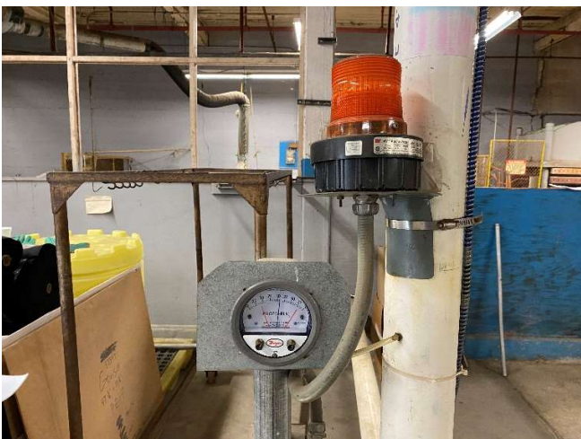
Photo 11. SSDS Gauge – 1.07" H 2 O vacuum.
