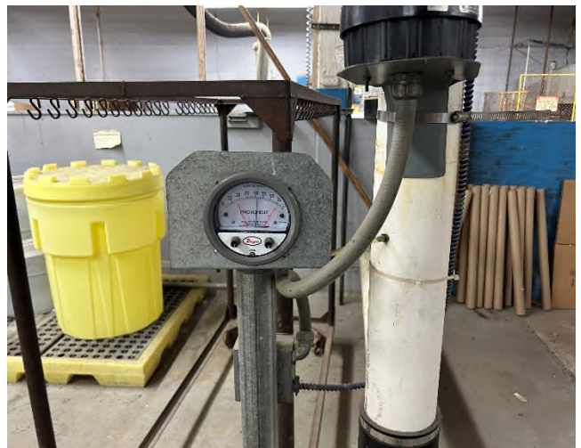
Photo 12. SSDS photohelic gauge, reading = 1.05'' H 2 O.
