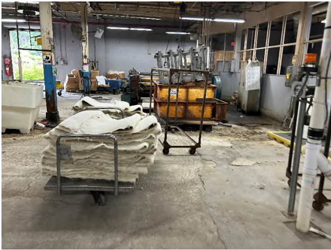
Photo 7. Piano Felt Bldg. floor (facing east).
