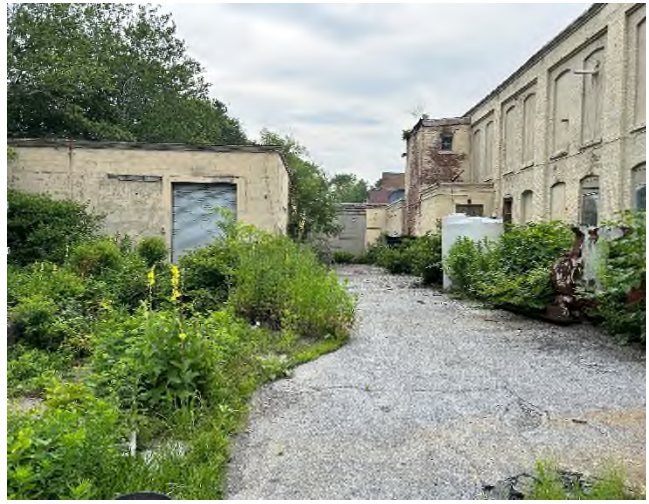
Photo 2. Southeast quadrant of Soil Mgt. Area (facing east).
