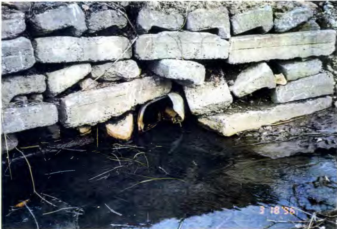
CULVERT BENT IN AND RESTRICTING FLOW
