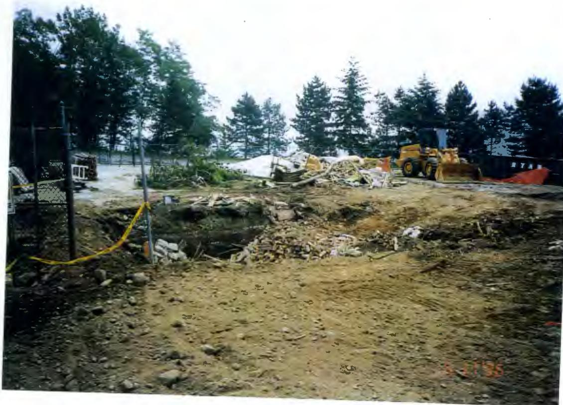
BACKFILLING THE BASEMENT WITH BRICK, CONCRETE
