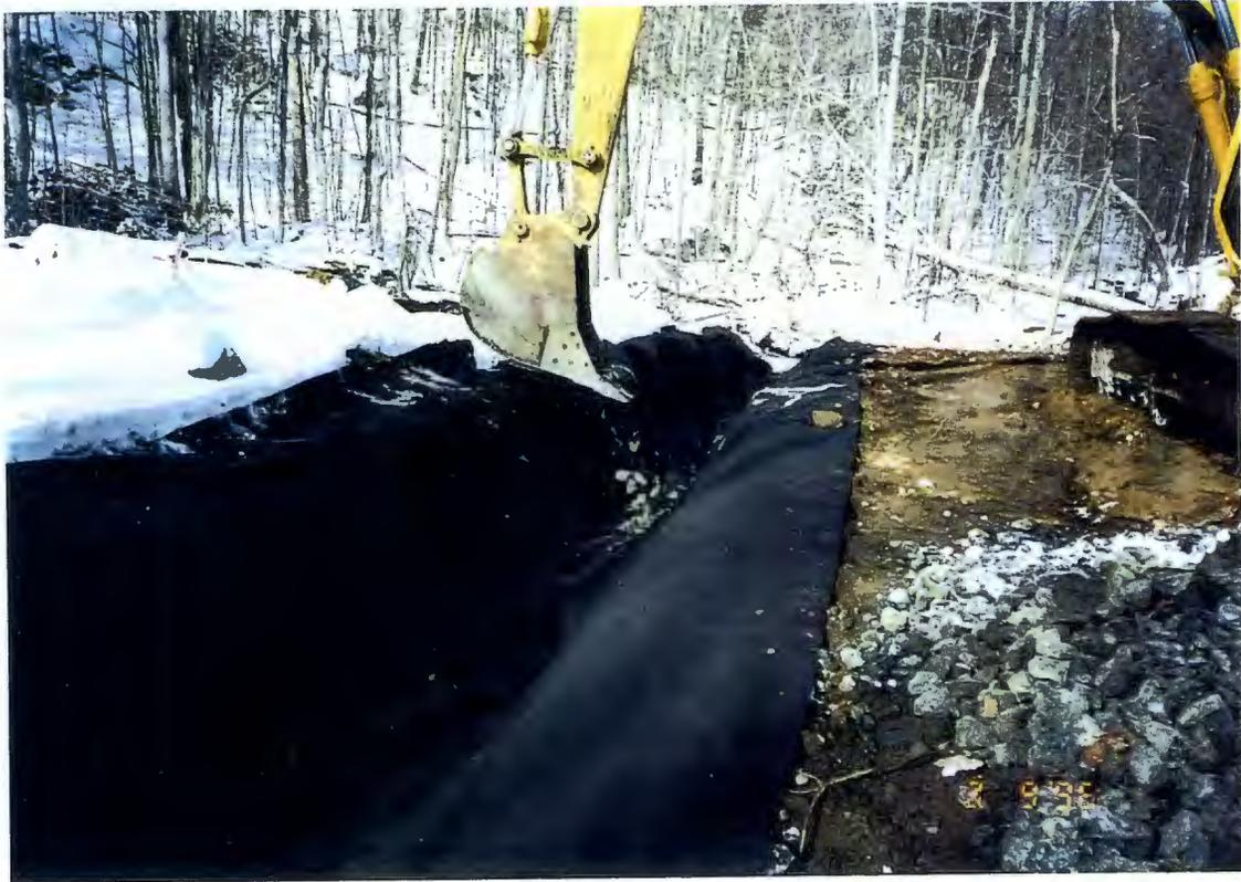
PLACING 6-12 INCH RIP RAP INTO GEOTEXTILE
