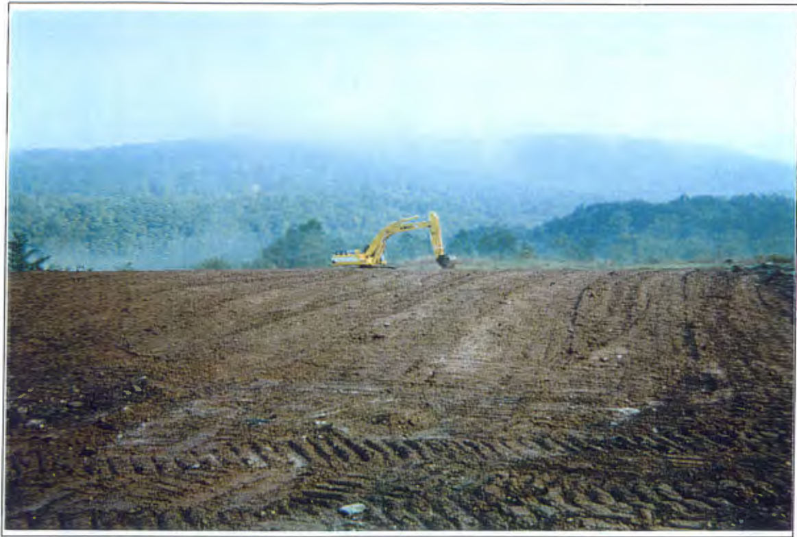
Cragston Landfill Replacement of Cragston Landfill cover
