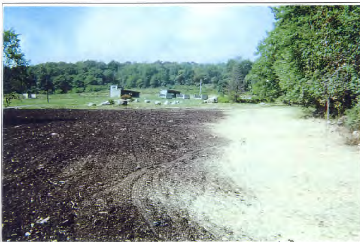
Village Farm Landfill Regraded Village Farm Landfill cover
