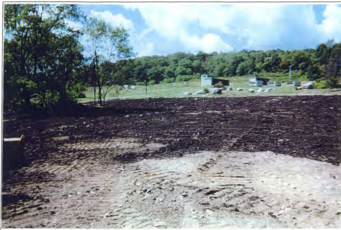
Village Farm Landfill Regrading Village Farm Landfill cover
