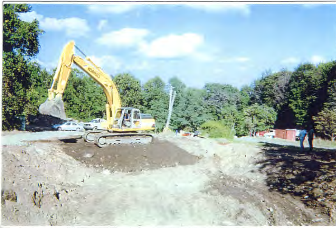
Village Farm Landfill Backfilling Village Farm Landfill excavation
