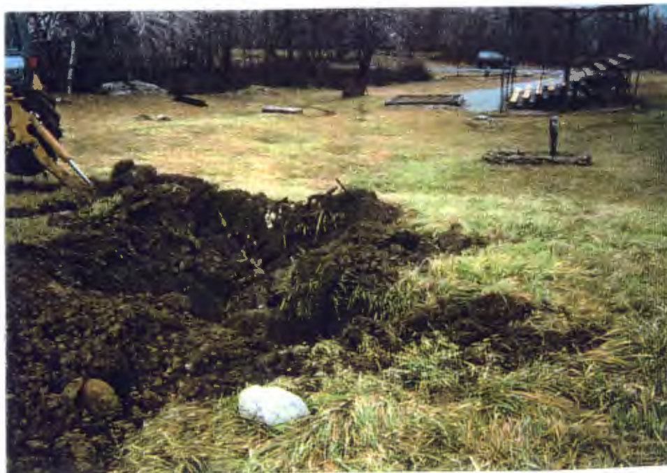
Photograph 4 Test Pit 03 - Landfill debris encountered Orientation - East
