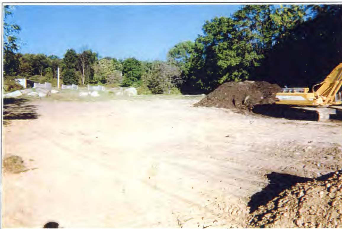
Village Farm Landfill Topsoil placement at the Village Farm Landfill
