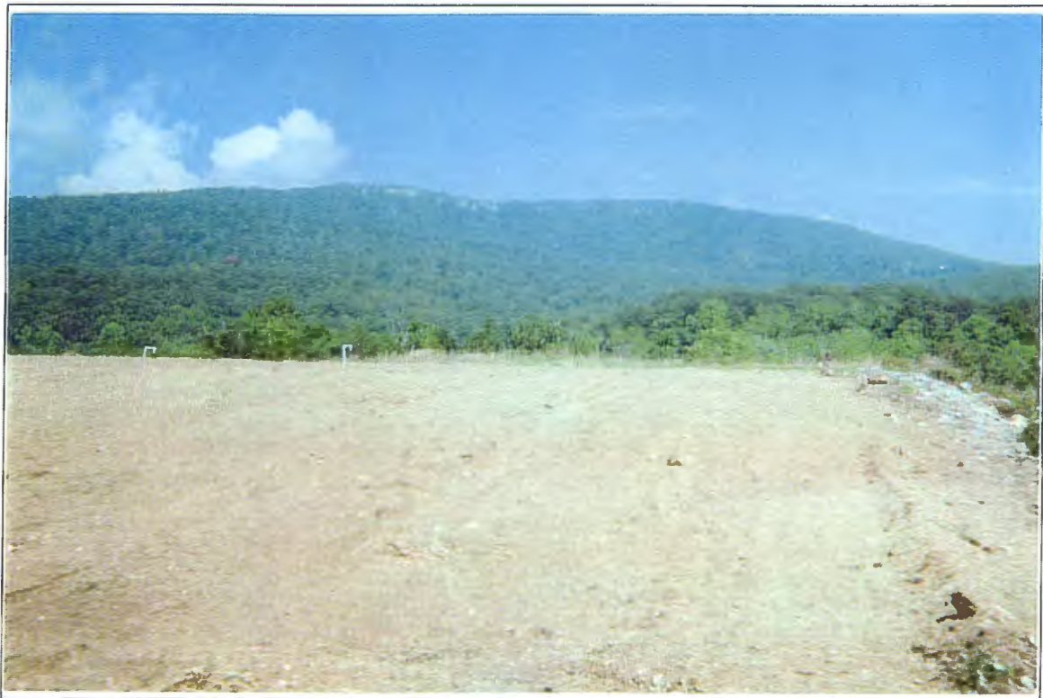
Cragston Landfill Regraded Cragston Landfill cover
