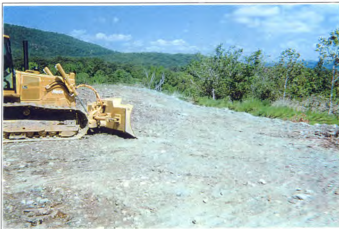
Cragston Landfill Regrading Cragston Landfill cover
