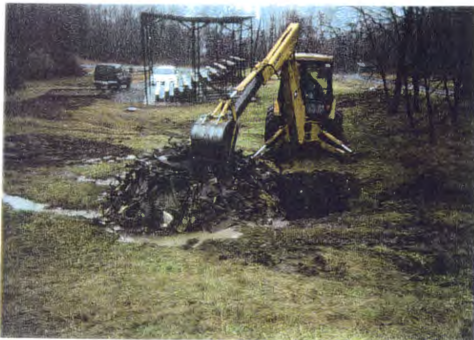
11 Test Pit 10 - Photograph 9 Landfill debris encountered to a depth of 12 ft., groundwater at 6 ft. Orientation - East
