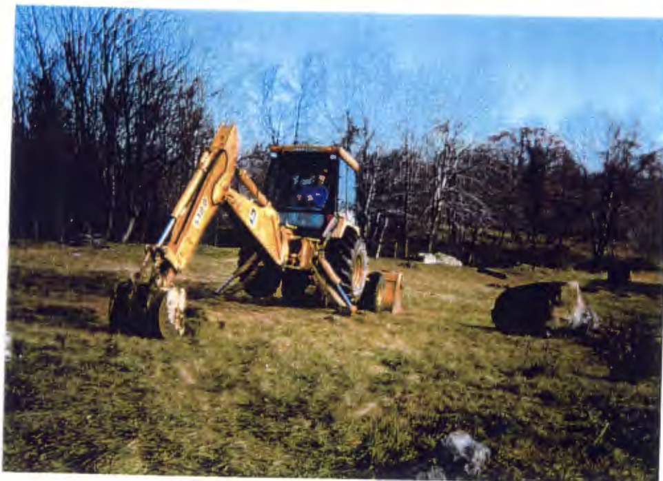
Photograph 1 Test Pit Survey at Village Farm Landfill Orientation - Northeast
