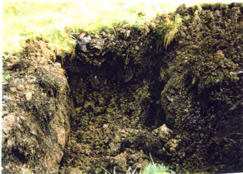
Photograph 5 Test Pit 04 - Landfill debris encountered
