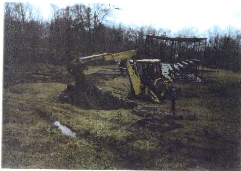
10 Test Pit 11 - Photograph 10 Landfill debris encountered to a depth of 12 ft., groundwater at 7.5 ft. Orientation - East
