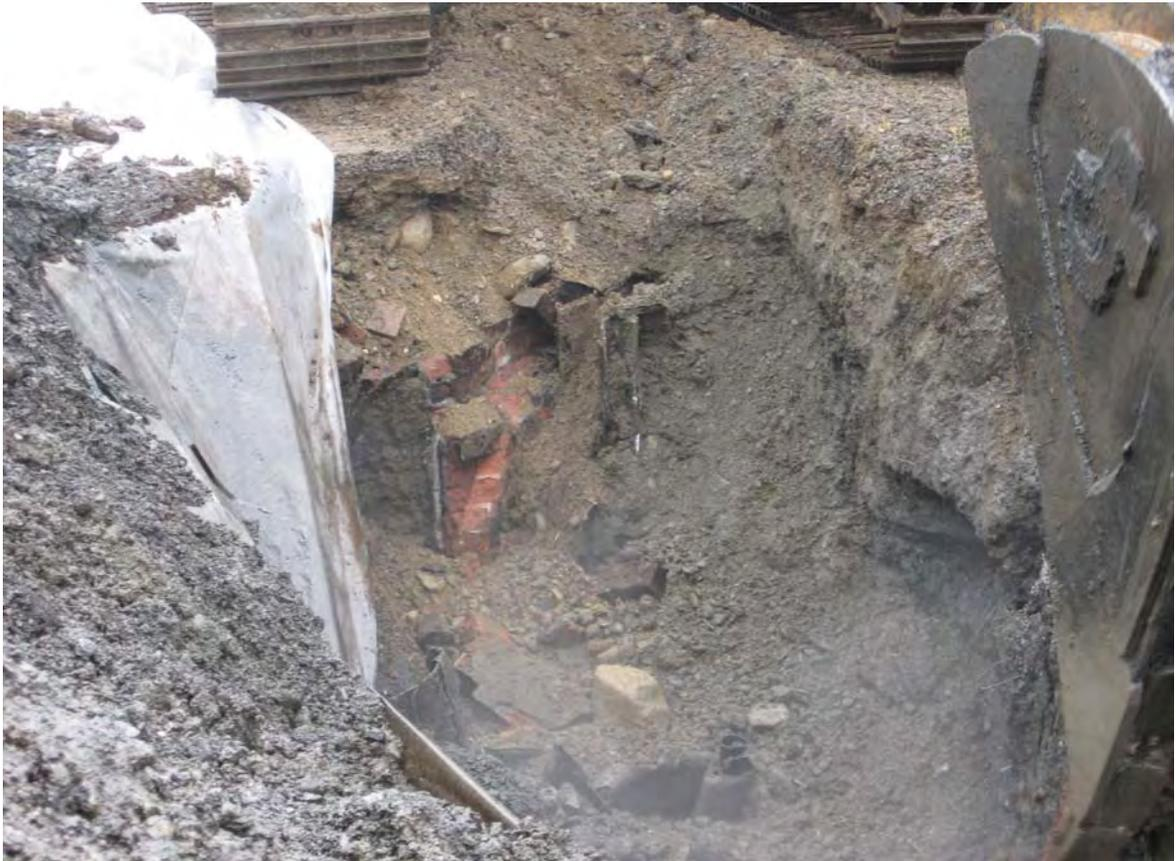
Photo 4: PDI-TP-5 facing north, former relief holder wall is exposed.
