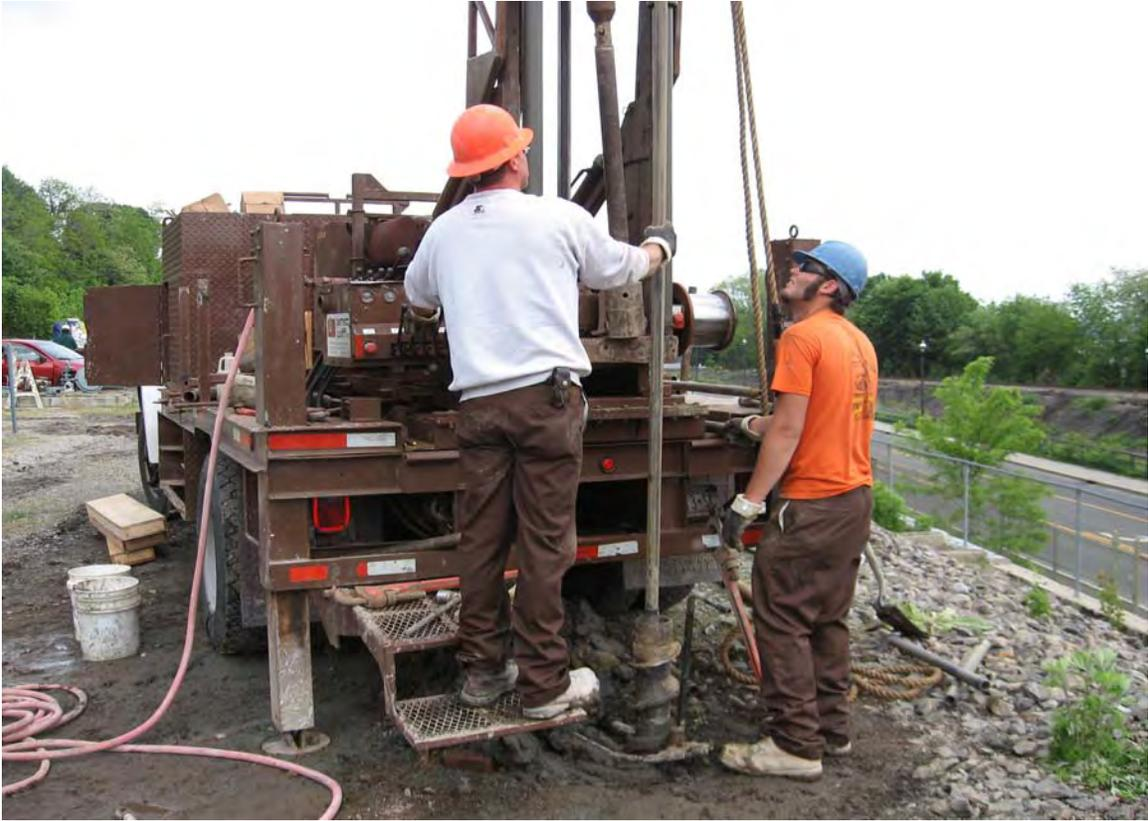
Photo 7: Hollow stem auger rig setup for sampling at soil boring PDI-SB-5.
