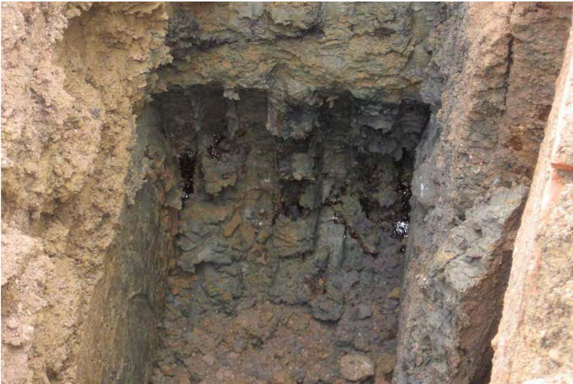
Photo 6: PDI-TP-4 NAPL pooling on water entering excavation at approximately 10' bgs.
